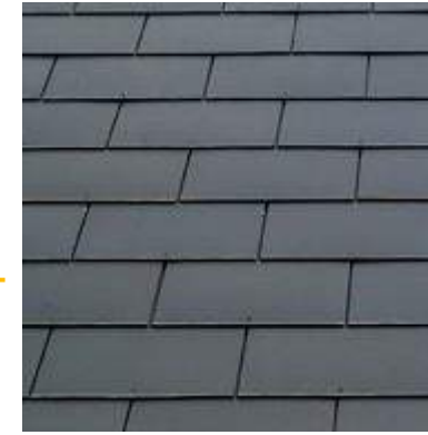
Fibre cement slate roof
