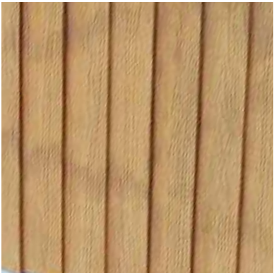
Fibre cement vertical cladding
