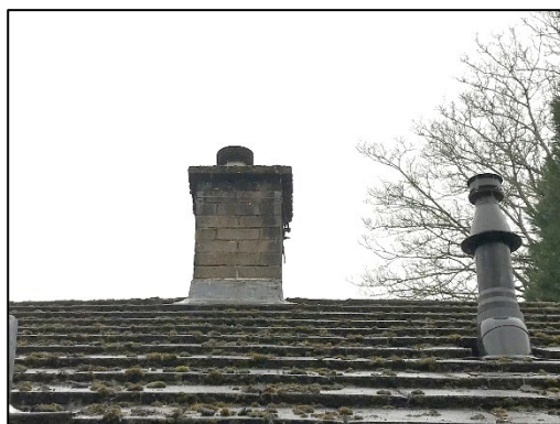
Figure 9: Brick chimney and plastic flue on northern elevation
