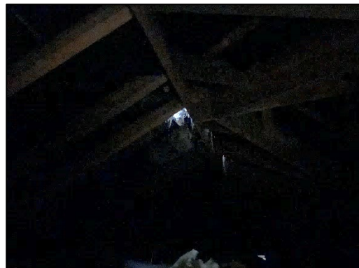
Figure 11: Light spill on the northern elevation
