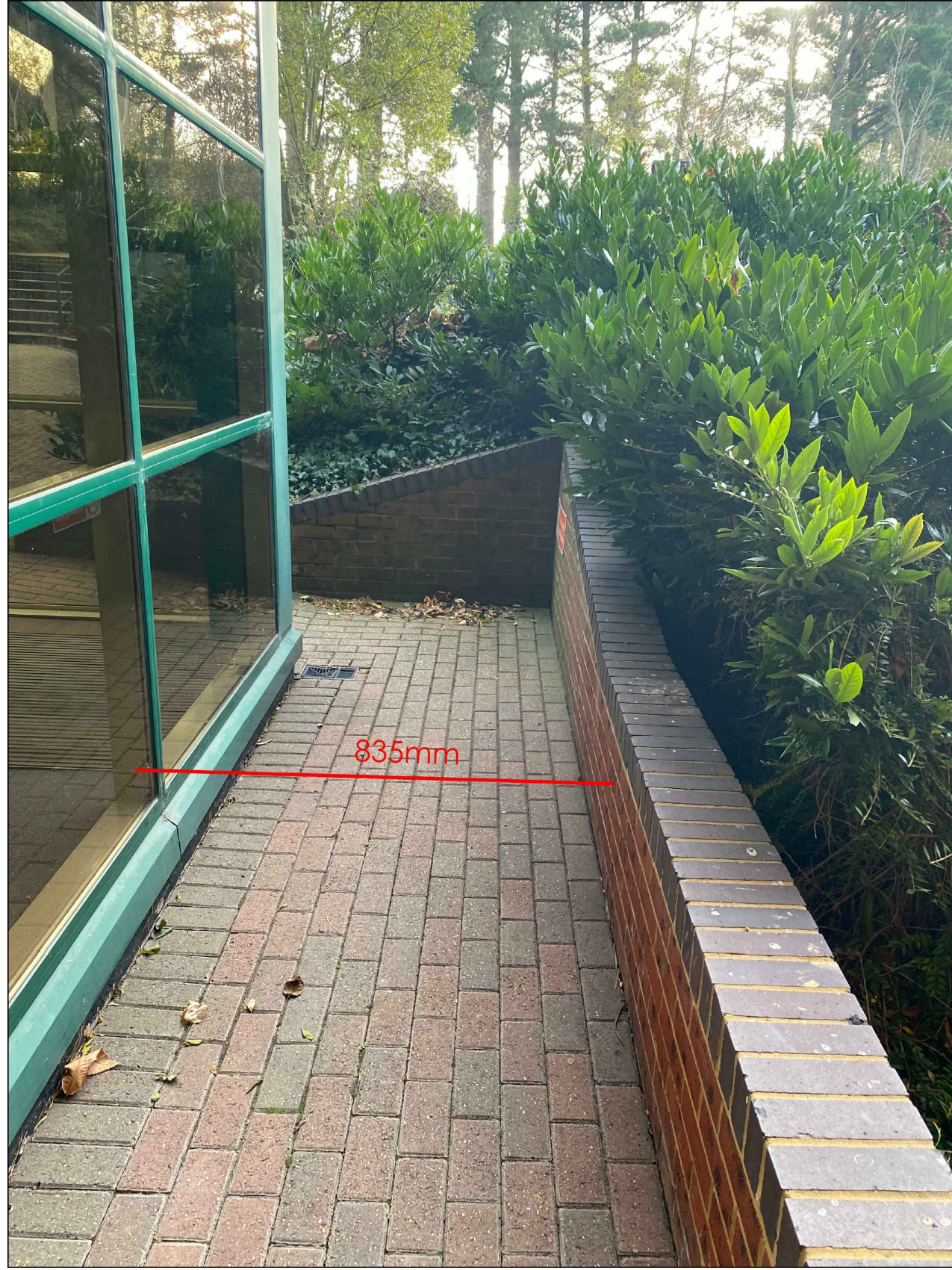
The proposed access will run on the outside the timber uprights and partially outside of the protection that is provided by the roof structure. the existing canopy is approx. 1800 from the external facade of the building meaning it would not fully cover the additional DDA ramp.
