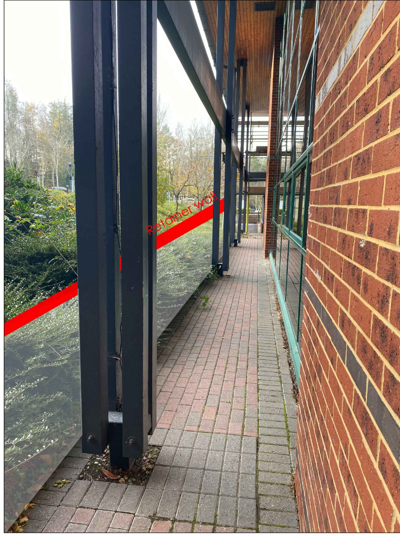
The existing staircase and walkway are surrounded by vegetation. to allow space for the DDA ramp and proposed walkway leading to the front entrance, the vegetation should be pushed back by 1200mm. A retaining wall can be used to support the soil laterally so that it can be kept at different levels on the two sides.
