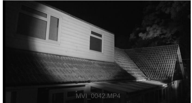
Photograph 46: NVA view of the east elevation at the end of the 2 nd dusk emergency survey
