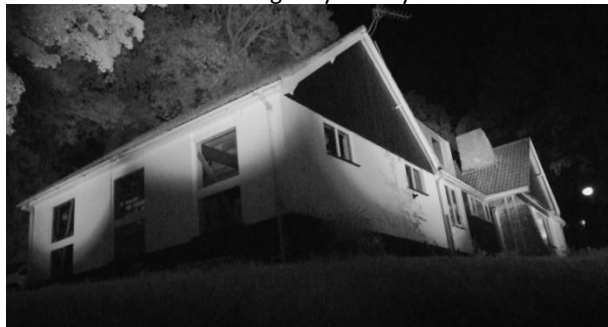
Photograph 43: NVA view of the north and west elevation at the end of the 1 st dusk emergency survey
