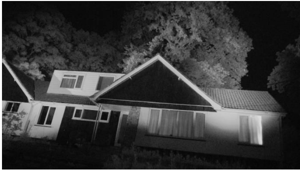
Photograph 45: NVA view of the west elevation at the end of the 2 nd dusk emergency survey
