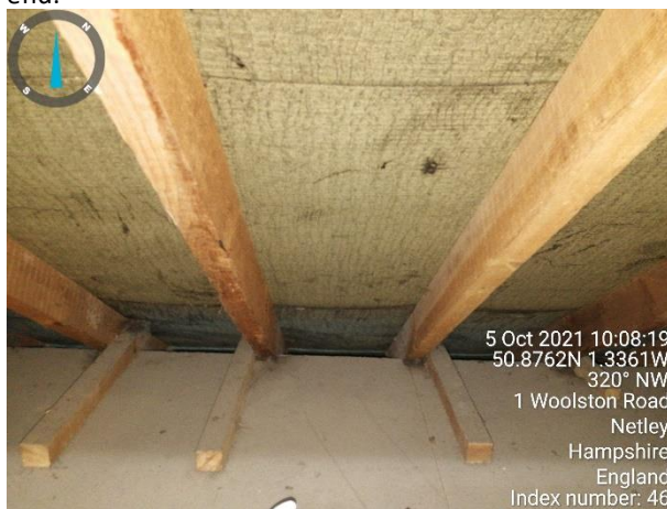
Photograph 3: Eaves on the northern length of garage loft with thin strip of light emitting.
