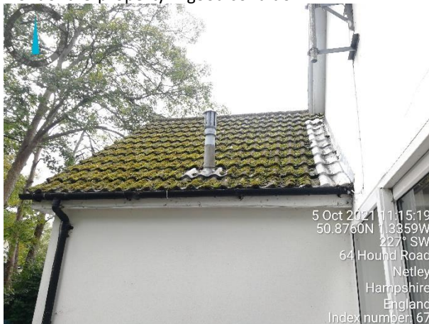
Photograph 21: View of single storey section located on the southern end with a moss-covered tiled roof.
