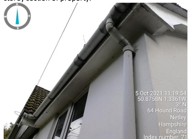
Photograph 24: View of wooden soffit on the southern end of the rear (west) elevation, in good condition.
