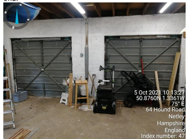
Photograph 4: View of ground floor of garage with two single garage doors.
