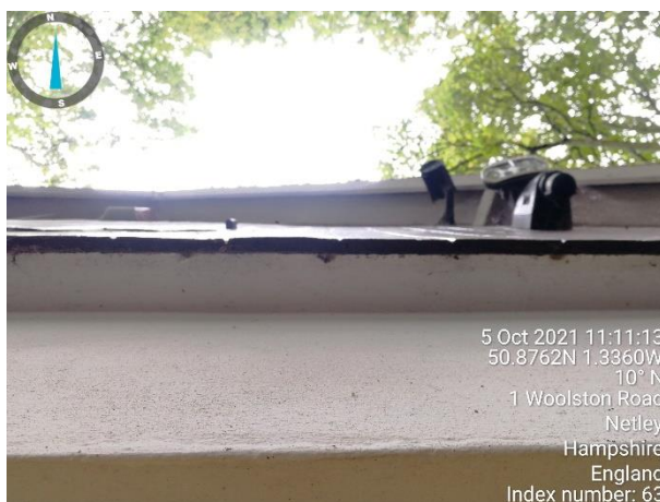
Photograph 17: View of the intact rendering behind the bottom run of shiplap at the front gable end of garage.
