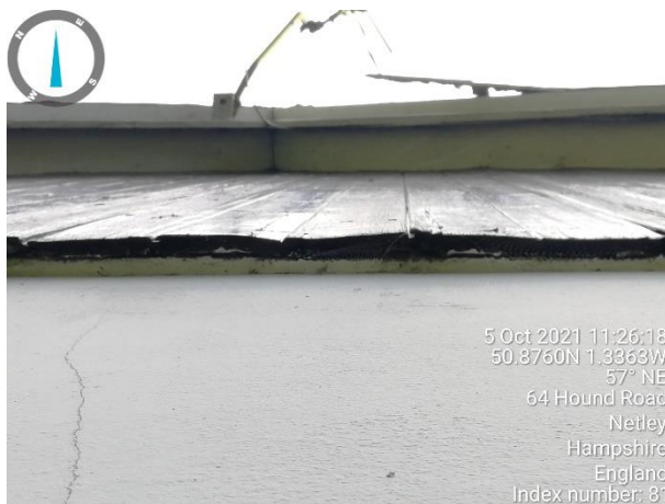
Photograph 33: View of lifting on the bottom of shiplap located on the garages western gable end.
