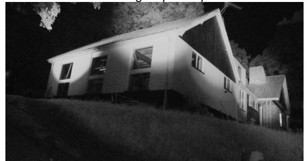
Photograph 44: NVA view of the west and north elevation at the end of the 2 nd dusk emergency survey
