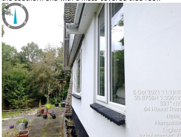
Photograph 23: View of the rendered rear section of property and patio to the left.
