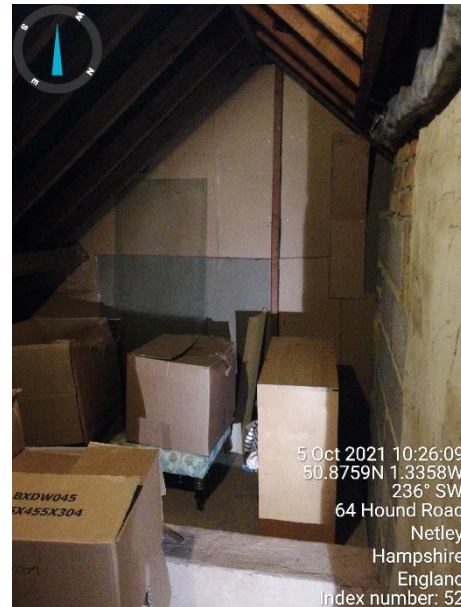
Photograph 8: View of southern loft with chimney to right.
