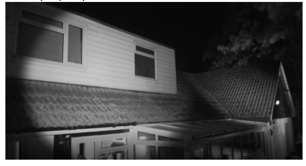
Photograph 42: NVA view of the east elevation at the end of the 1 st dusk emergency survey
