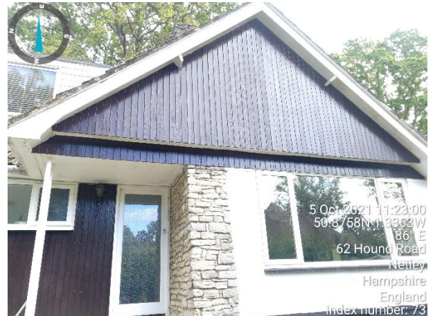
Photograph 26: View of shiplap gable end to the rear of the property with rendered and stone facing.
