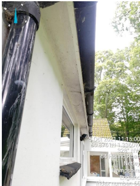
Photograph 19: View of the wooden soffit along the front of the property in good condition.
