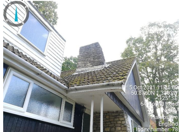
Photograph 30: View of the chimney and porch to the rear of the property.
