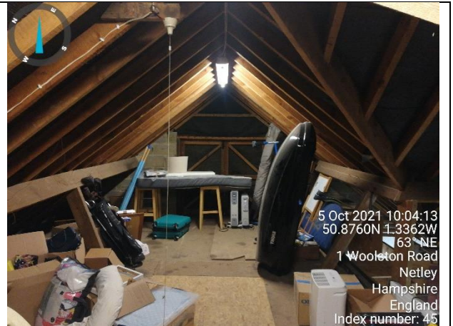
Photograph 2: Loft above garage looking at east gable end.
