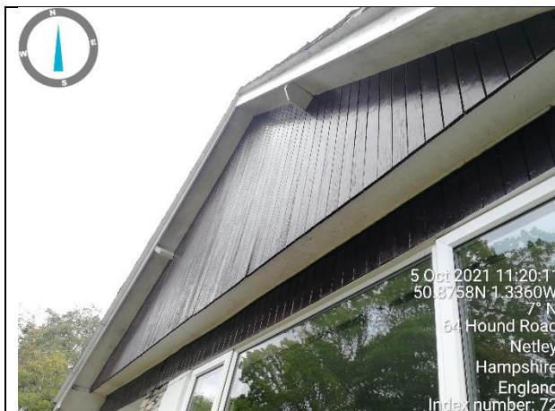
Photograph 25: View of the shiplap gable end with wooden soffit box in good condition located on the rear of the property.
