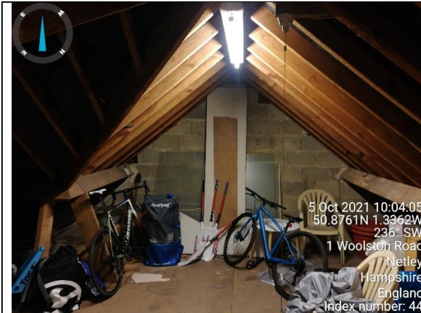
Photograph 1: Loft above garage looking at west gable end.
