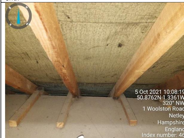
Photograph 3: Eaves on the northern length of garage loft with thin strip of light emitting.
