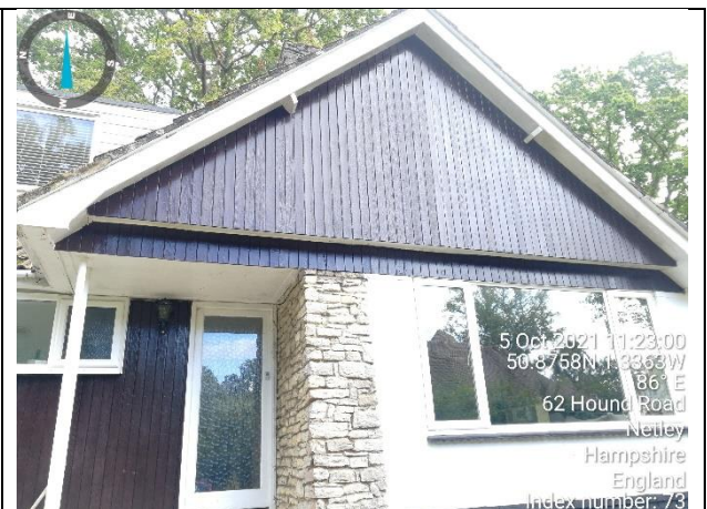
Photograph 26: View of shiplap gable end to the rear of the property with rendered and stone facing.
