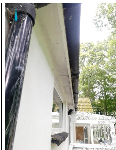
Photograph 19: View of the wooden soffit along the front of the property in good condition.
