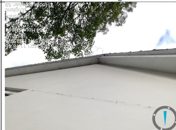
Photograph 20: View of the southern gable end with rendered walls and wooden soffit in good condition.
