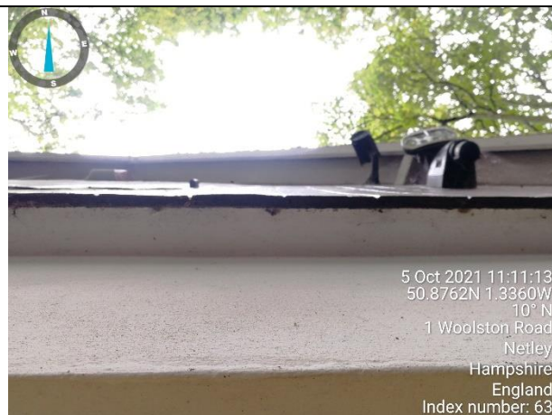
Photograph 17: View of the intact rendering behind the bottom run of shiplap at the front gable end of garage.
