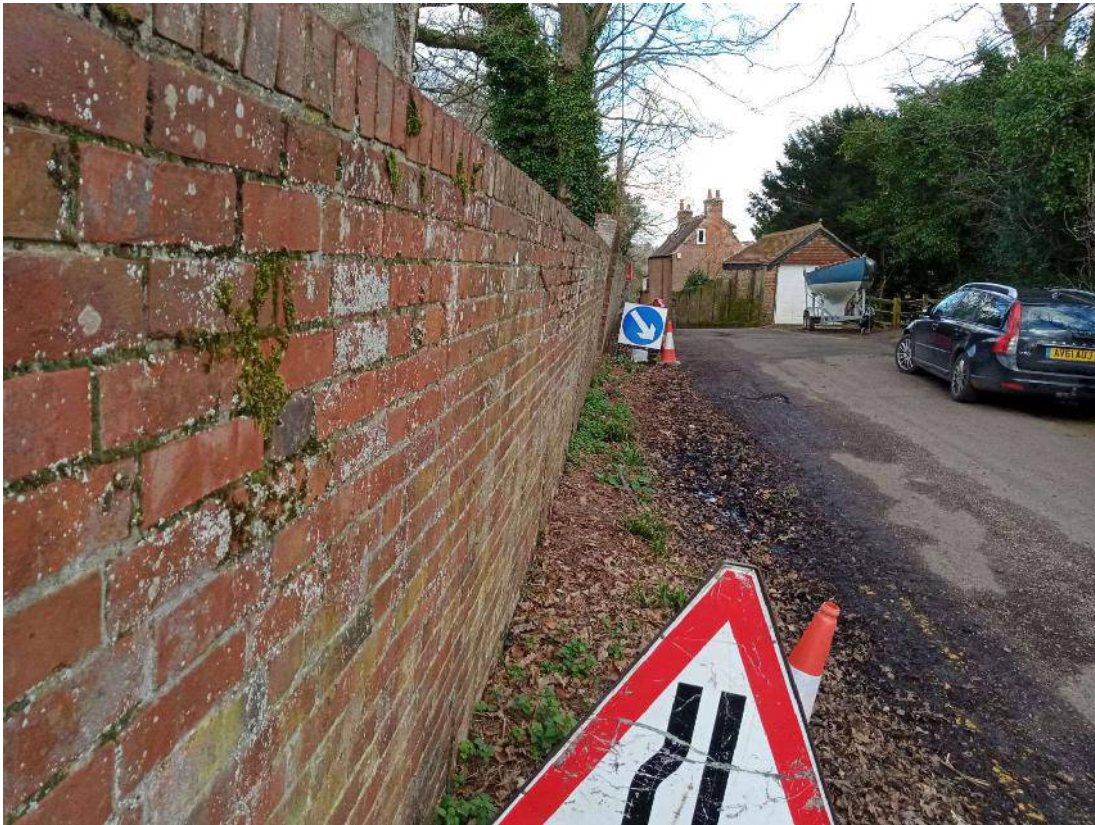
Photograph 3 – View along wall Length A
