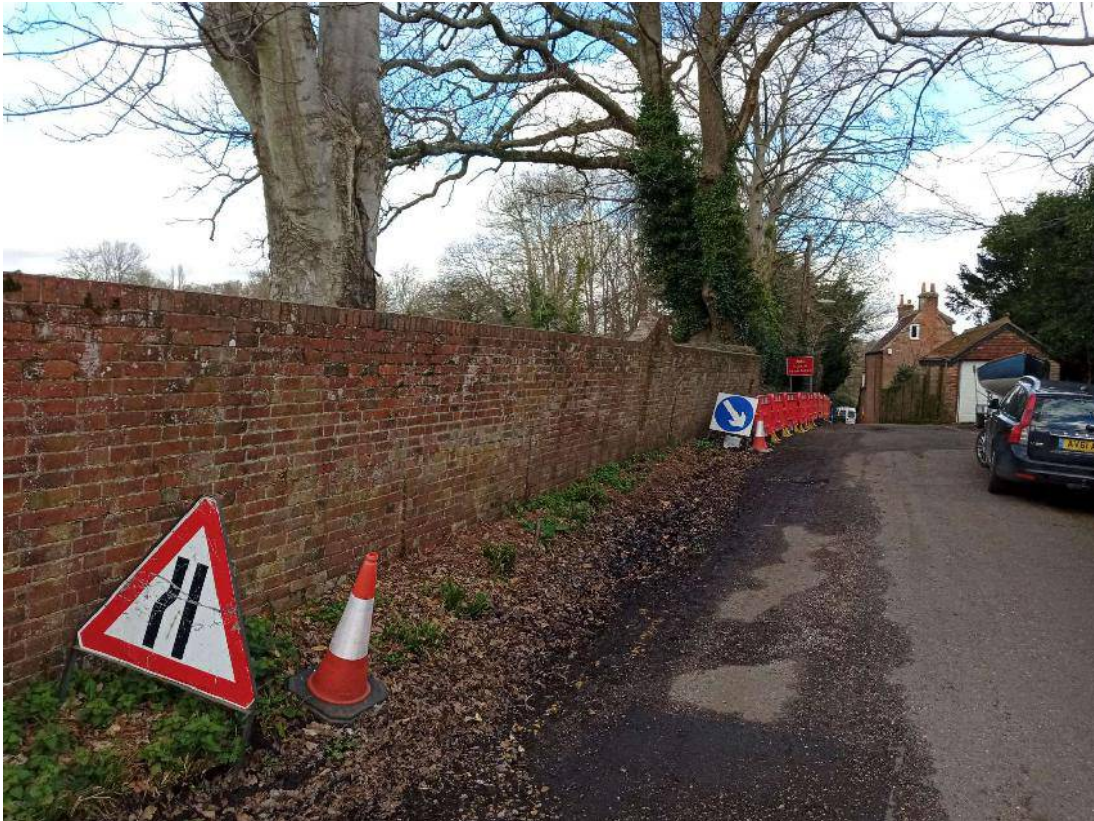
Photograph 2 – General view of wall Length A
