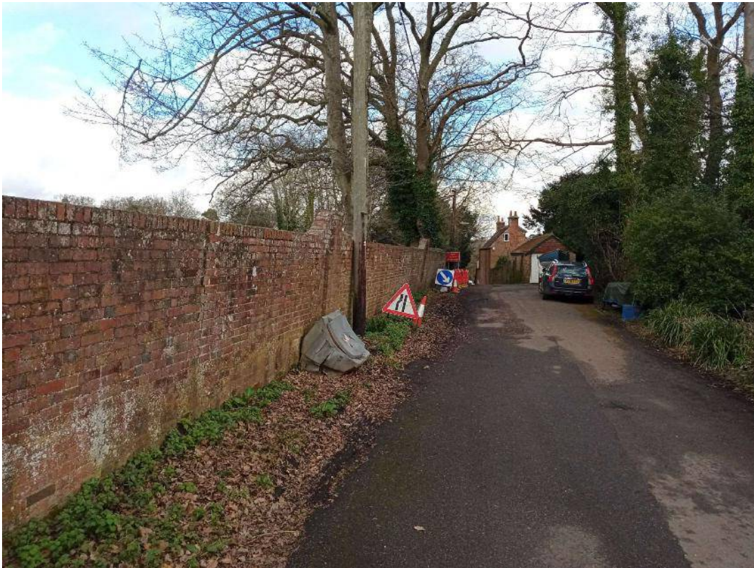
Photograph 1 – General view of Southern end of wall
