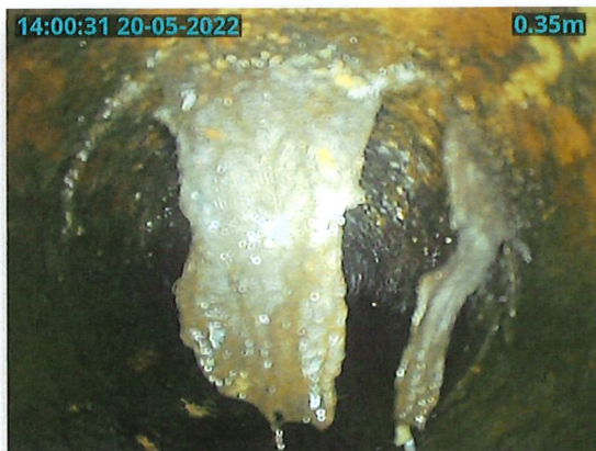
Fig 1.1: This shows the root ingress located within the SVP pipework.
