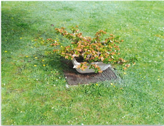
Fig 2.1: This shows the manhole located at the front of the customers property.
