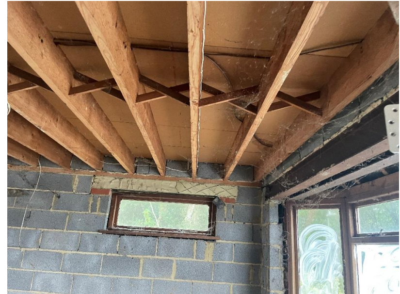
B1 – open window on ground floor
