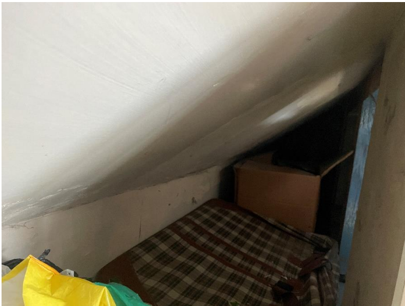
B1 – well-sealed internal cupboards at southern extent
