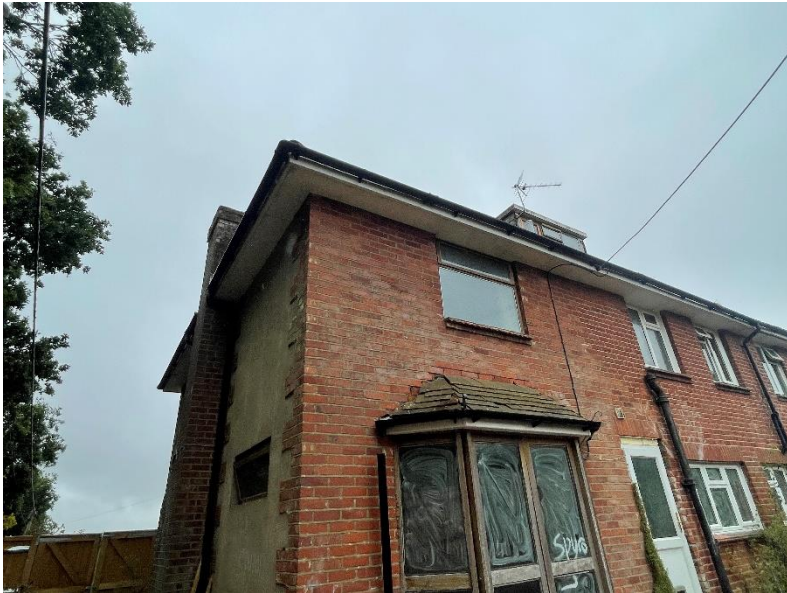
B1 – northern and western elevations
