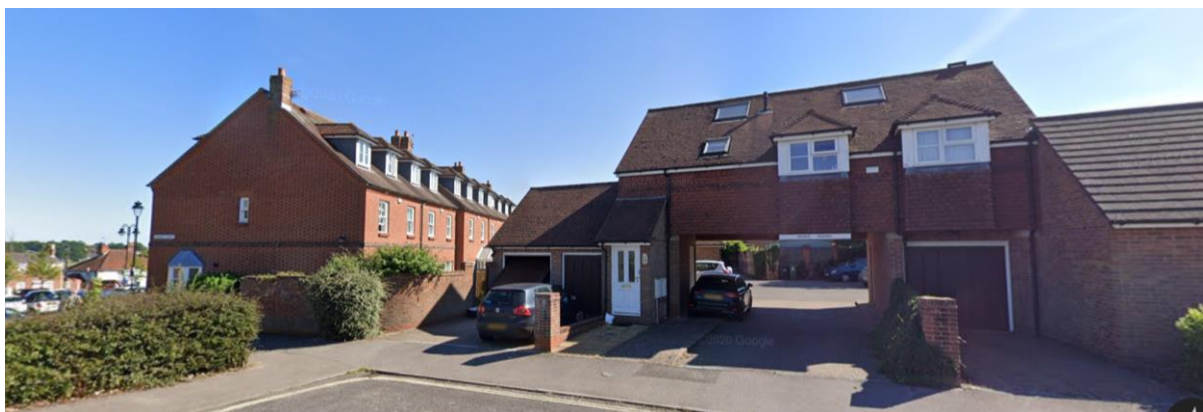
Figure 5 Residential Development located to the South of the Application Site
