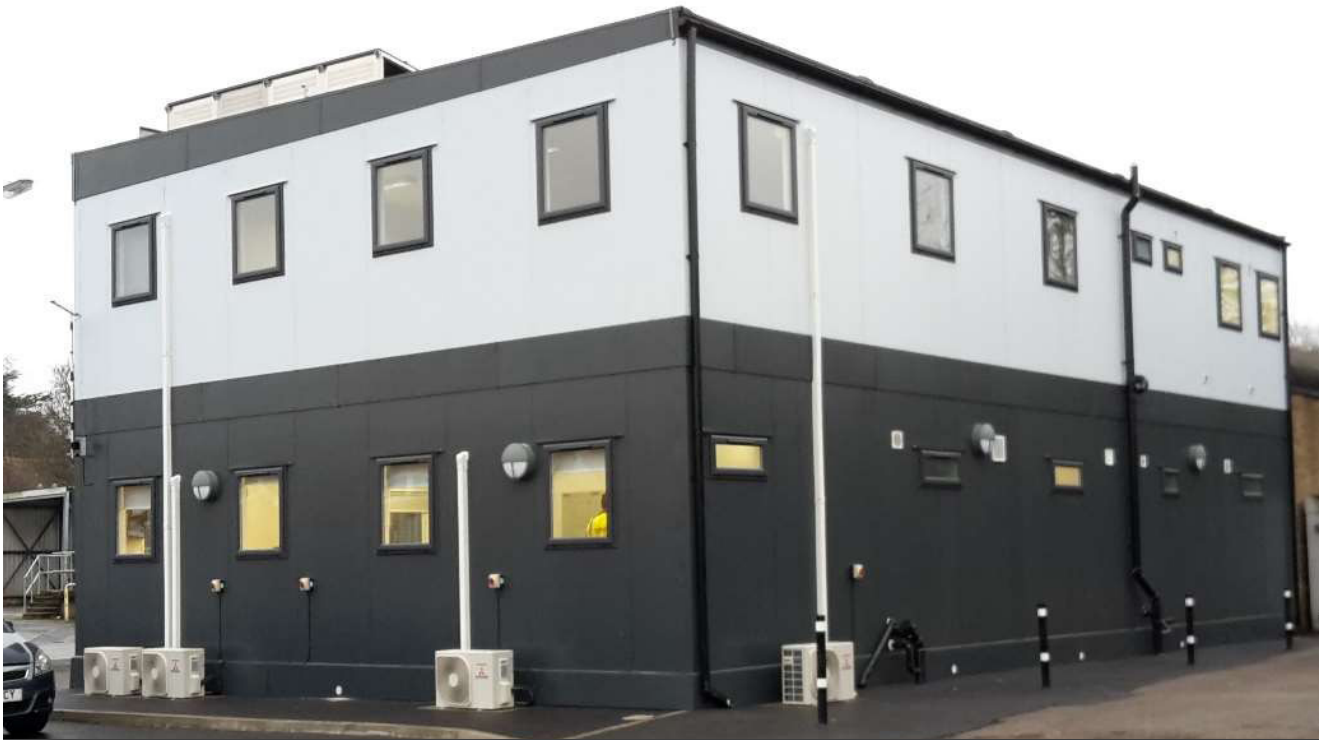
Figure 7: Example of a modular building facade - Gedling Borough Council, Jubilee Waste Collection Centre
