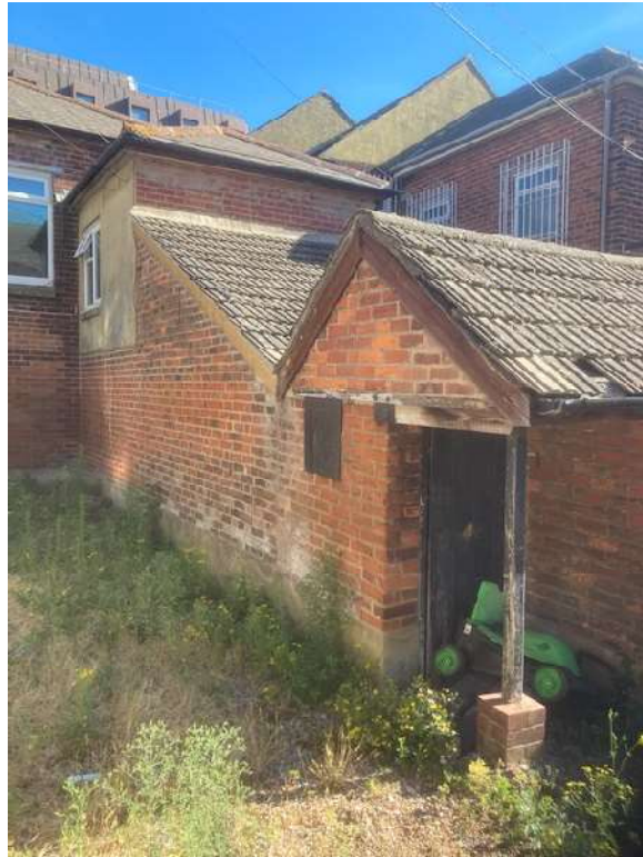
Fig.4 – Photograph showing the various extensions on the rear part of the building at 5 Leigh Road.
