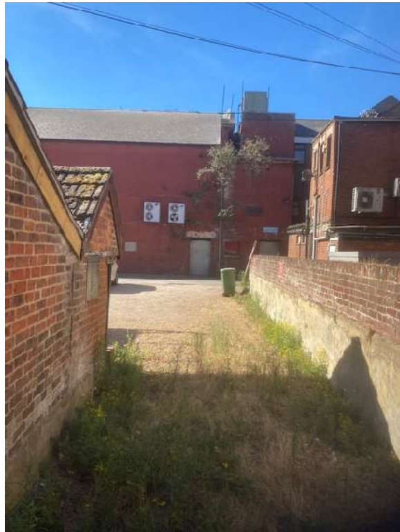
Fig.5 – Photograph looking south from the rear of the main part of the building at 5 Leigh Road.
