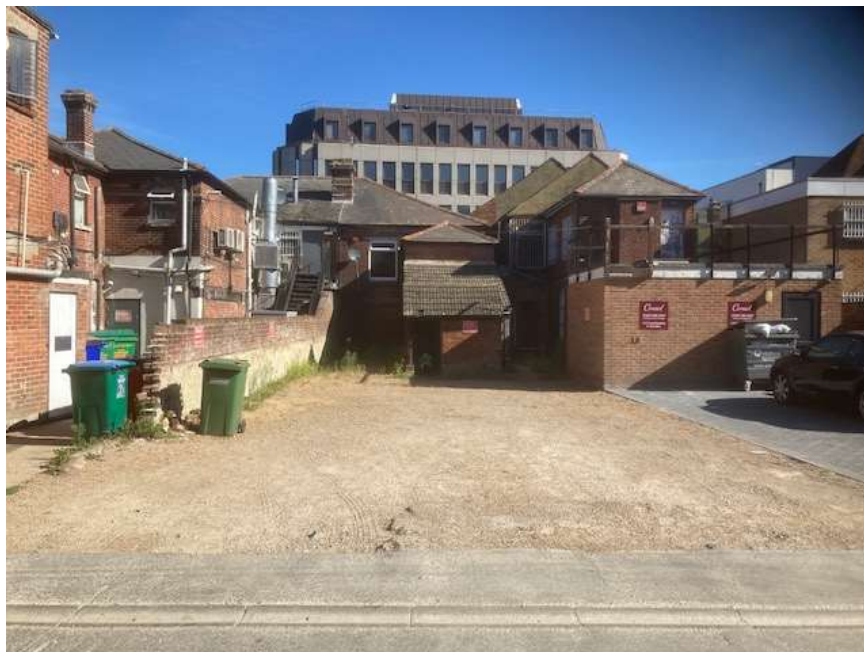
Fig.1 – Photograph showing the south (rear) elevation of 5 Leigh Road (centre) from Mitchell Road with the large area of hardstanding in the foreground.
