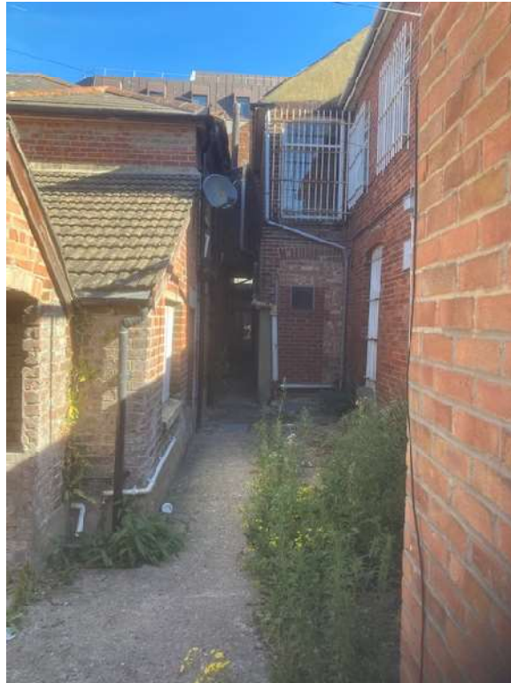
Fig.6 – Photograph taken from the back of the building at 5 Leigh Road looking towards the passageway between 5 and 7 Leigh Road (right).
