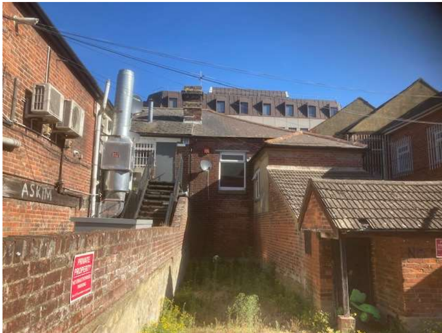
Fig.3 – Photograph showing the various extensions on the rear part of the building at 5 Leigh Road with the existing brick boundary wall (left).
