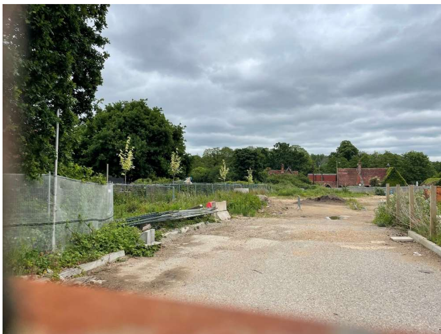
Looking through a gap in the hoarding into the site
