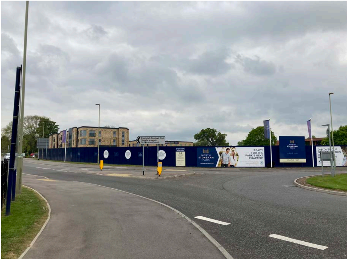
Plate 1: View of hoarded study site from adjacent roundabout
