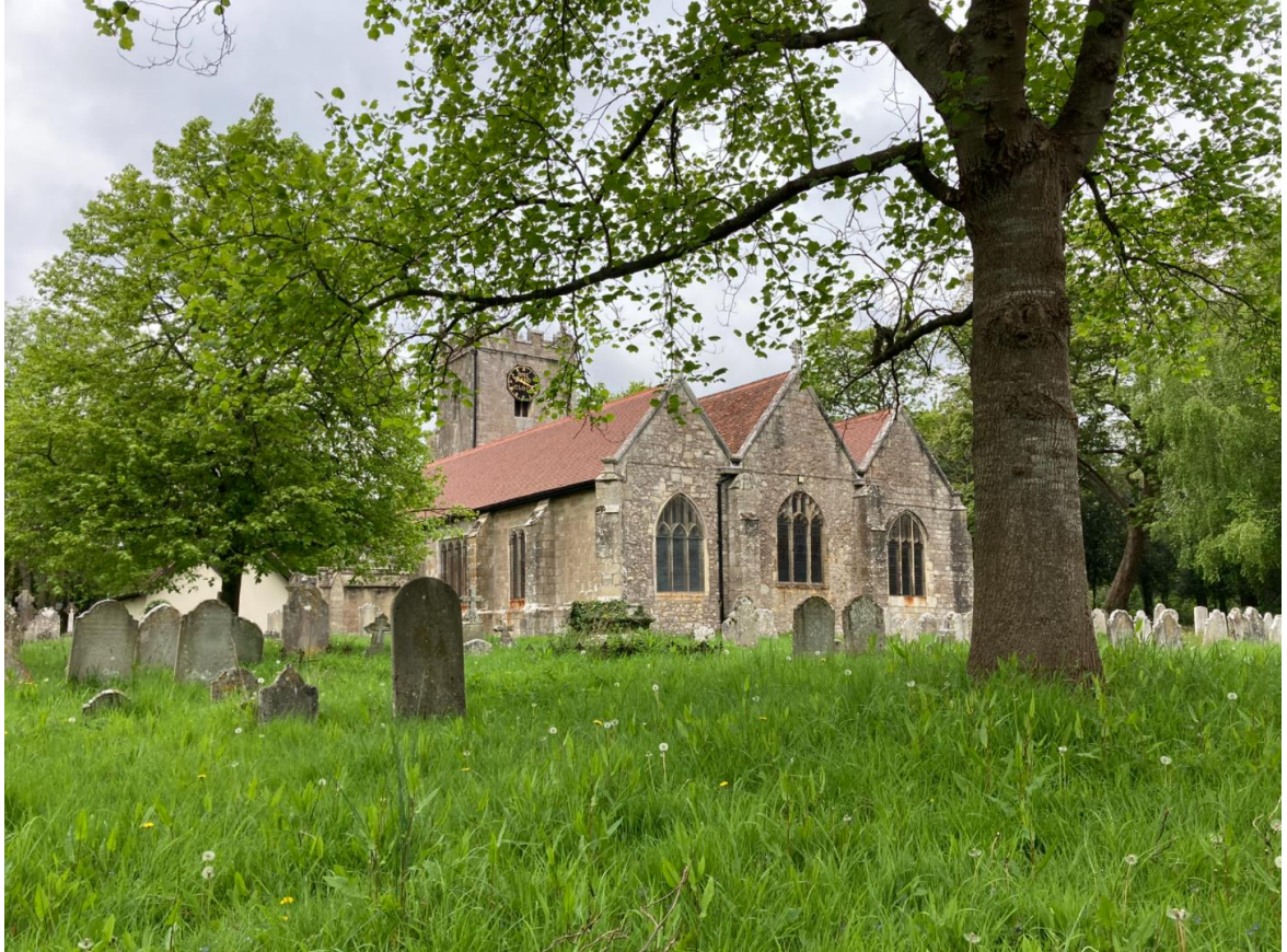
Figure 17 St Nicolas Church viewed from Stoneham Lane
