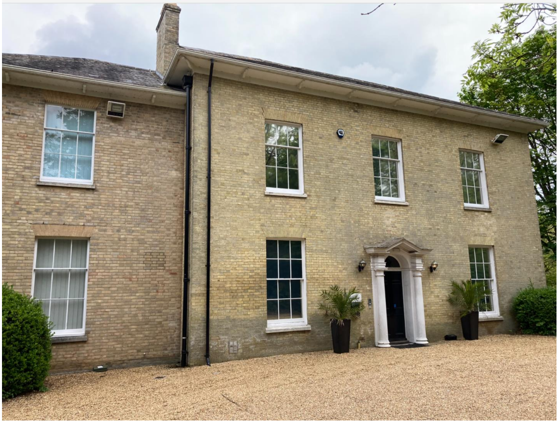
Figure 19 The Old Rectory west elevation seen from within the Business Complex
