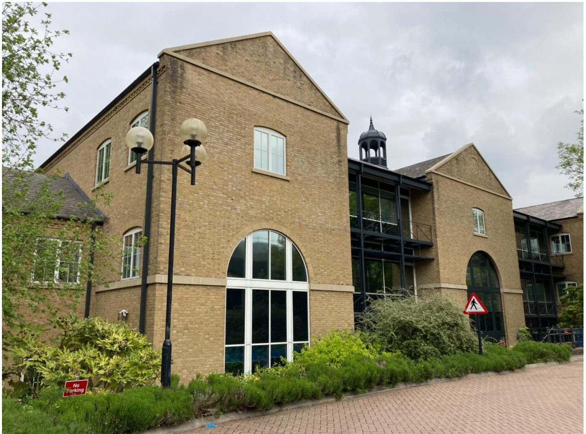
Figure 21 View from the Old Rectory towards the Site
