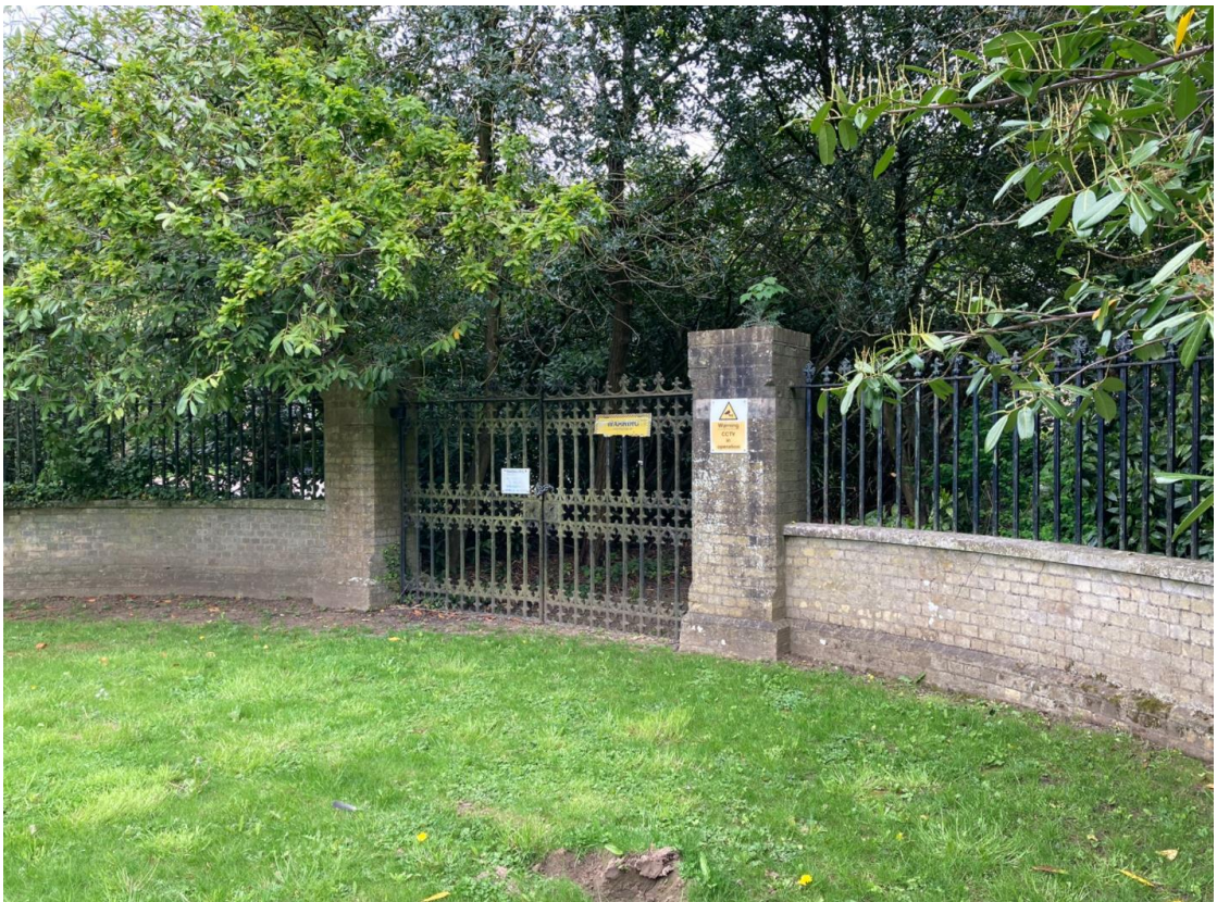
Figure 20 The Entrance Gates to the Old Rectory viewed from Stoneham Lane
