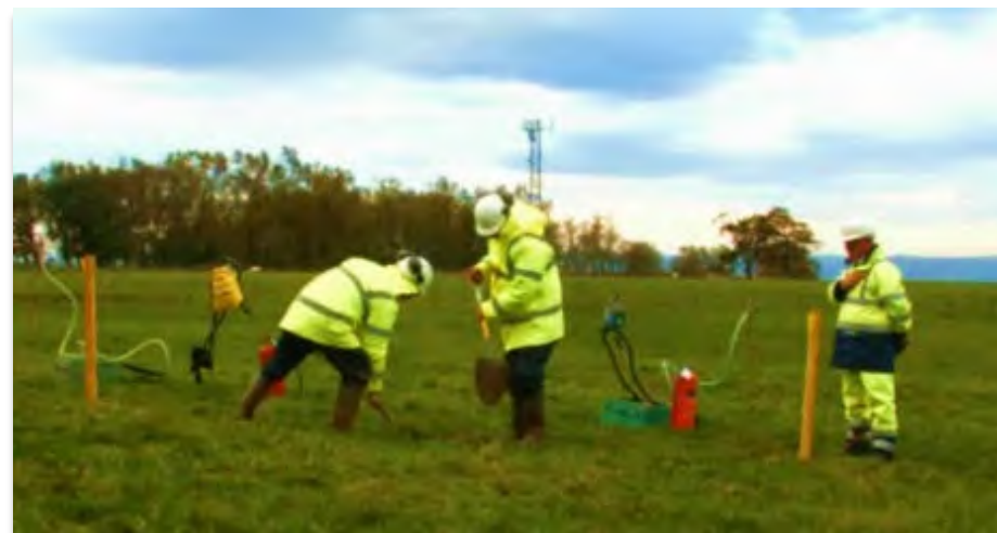
Figure 4. Hand Excavated Trial Hole
