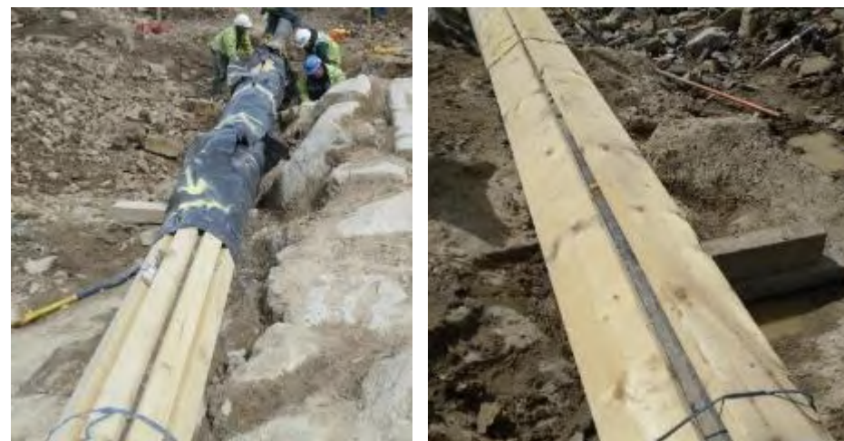
Figure 14. Protective cladding applied to pipeline
