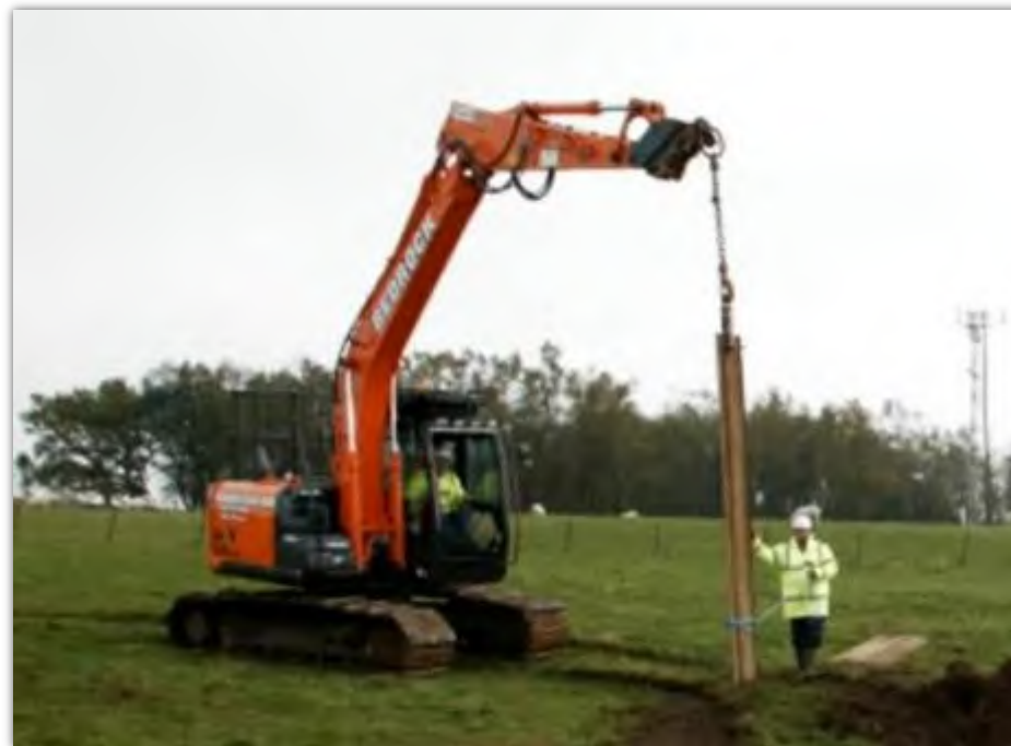
Figure 21. Example Lifting Operation
