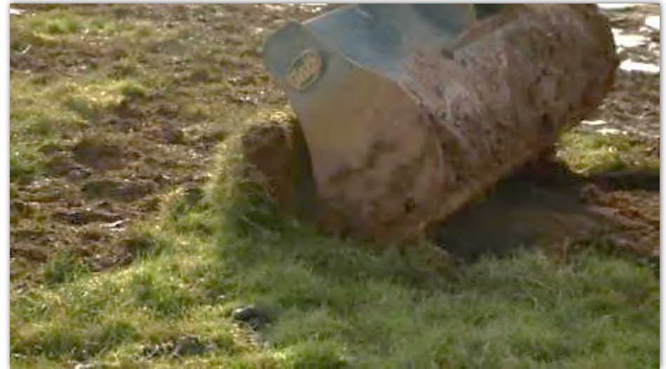
Figure 12. Top Soil Stripping
