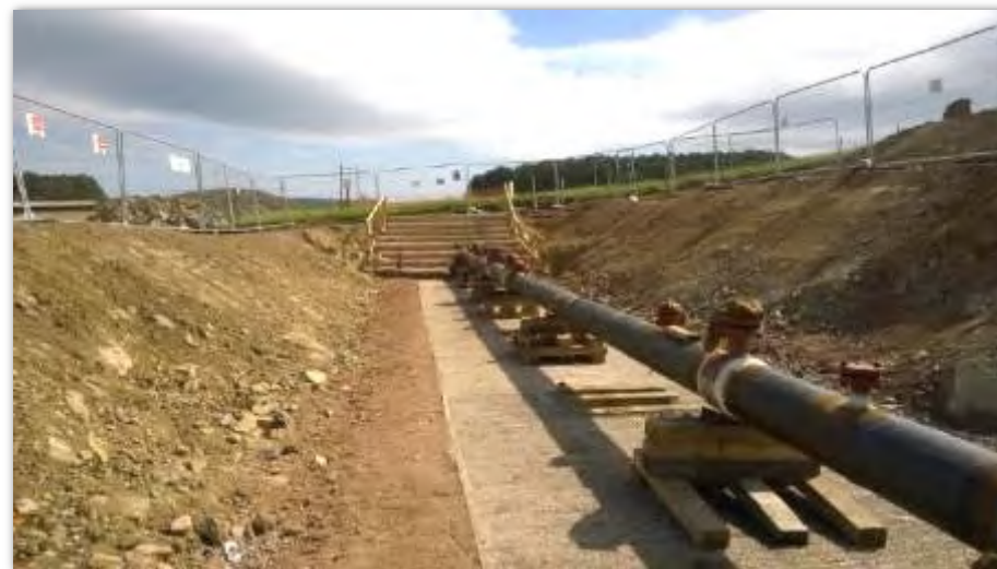
Figure 20. Pipeline Supports
