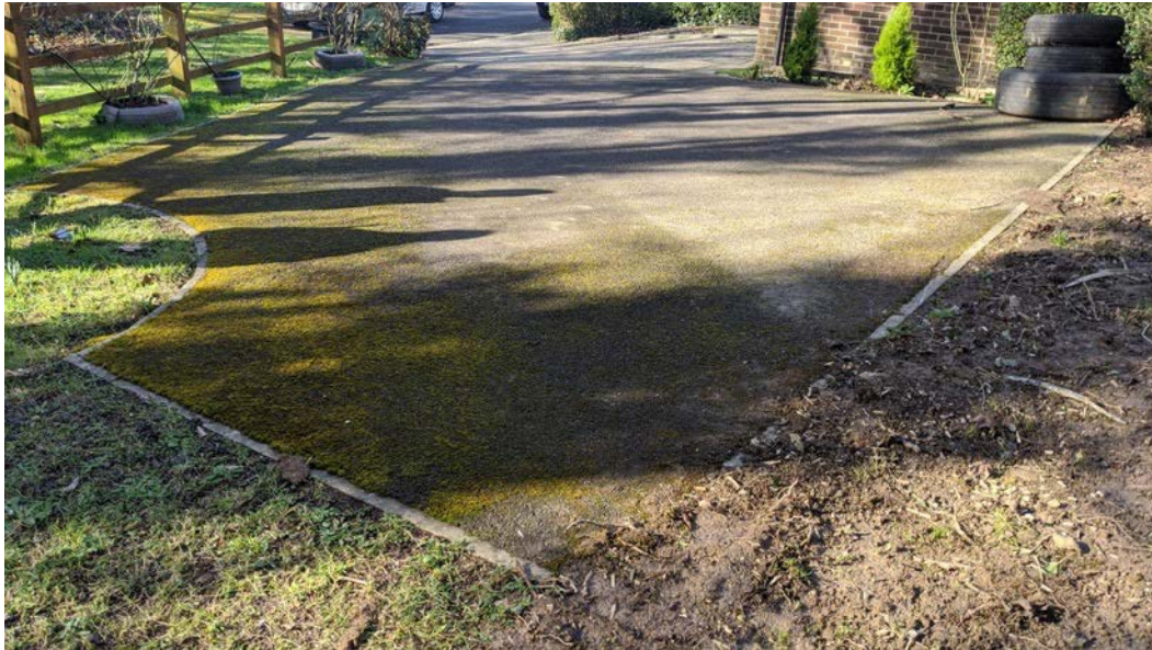
Figure 6. Hard standing driveway at the South entrance to the site (February 2022).
