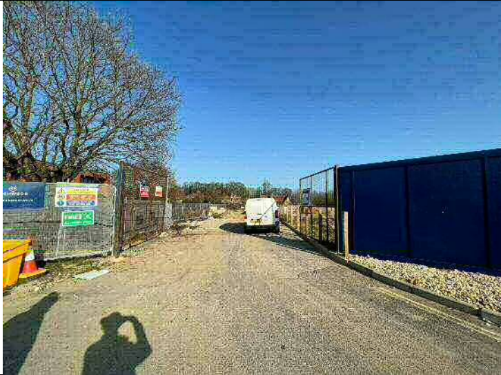
Photograph 1 – A view of the site entrance in the north-west corner.
