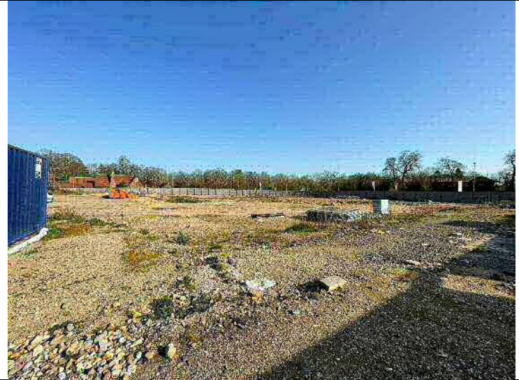
Photograph 2 – A view south across the site.
