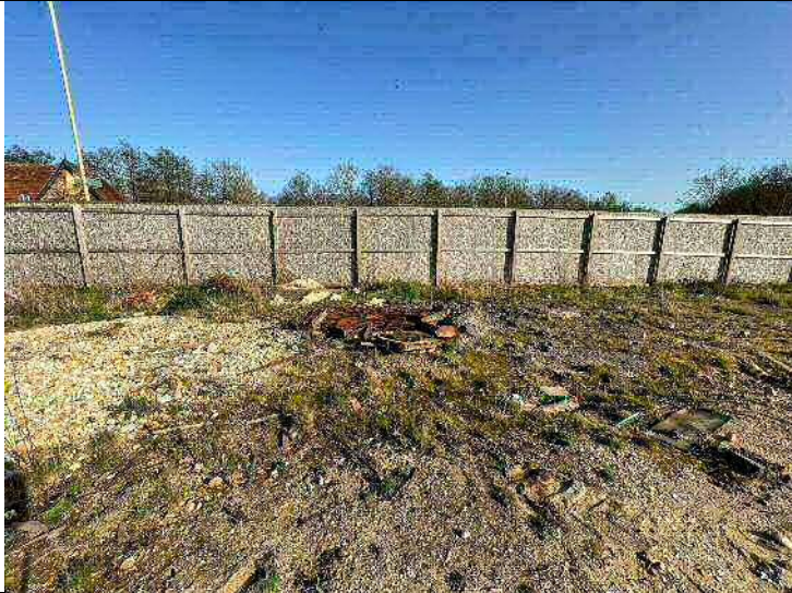
Photograph 5 – A view of the burnt waste materials on-site.
