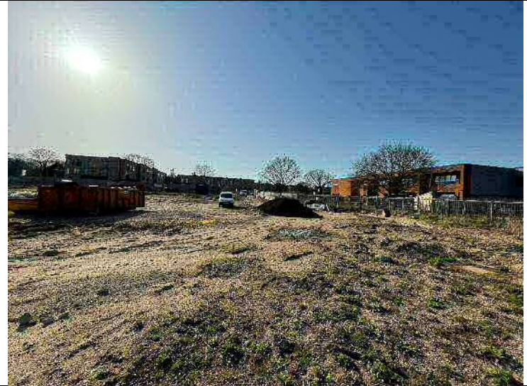
Photograph 6 – A view of the stockpile in the northern area of the site.
