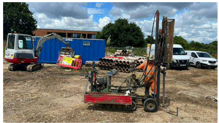
Photograph 2 – A view of some of the plant and materials being stored on site during the supplementary investigation.
