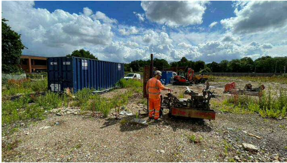
Photograph 1 – An example of the rig on position.
