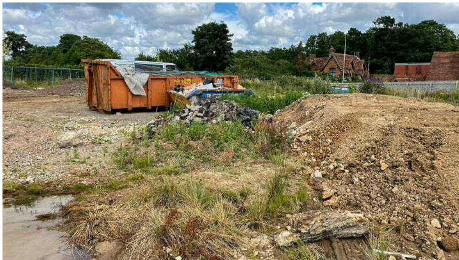
Photograph 3 – A view of the excavated materials from off-site works being stockpiled on site during the supplementary investigation.
