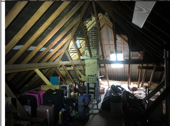
Internal loft space showing roof light/velux window
