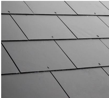
Artificial Slate Roof Tiles on both the buildings.
