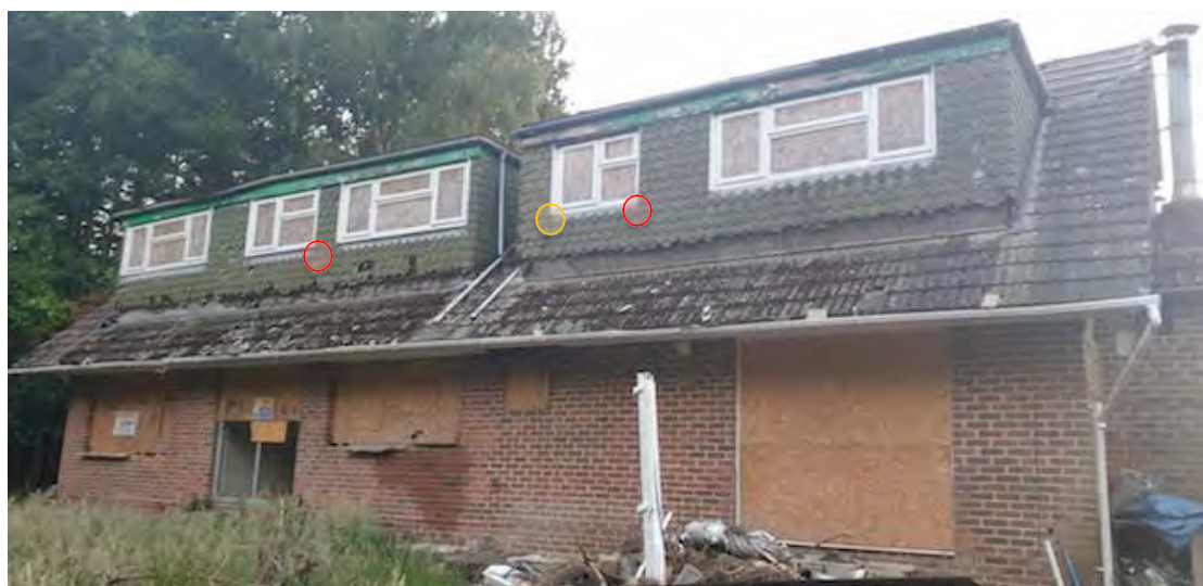
Figure 28. Approximate locations of individual Common Pipistrelle emergences (Red dot) and 4 Common Pipistrelle and 1 Soprano Pipistrelle (orange dot) on the south east facing aspect of the dwelling.
