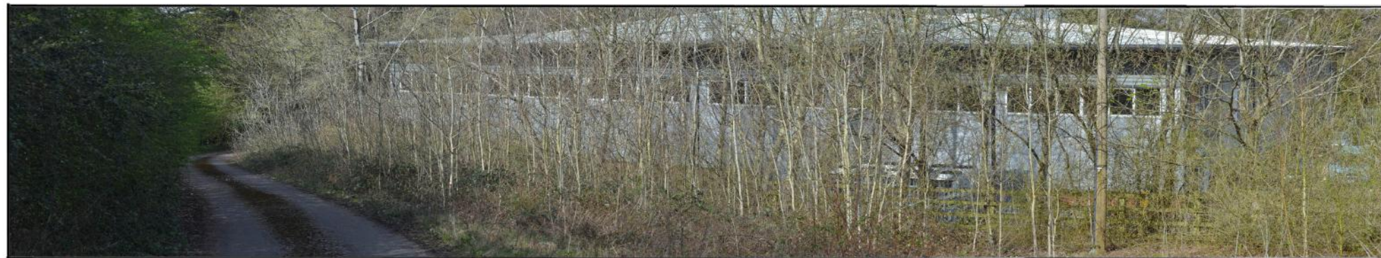
Viewpoint D Date: 30th March 2021. OS grid ref: SU 48200 14337. From the site access track viewing north-east
