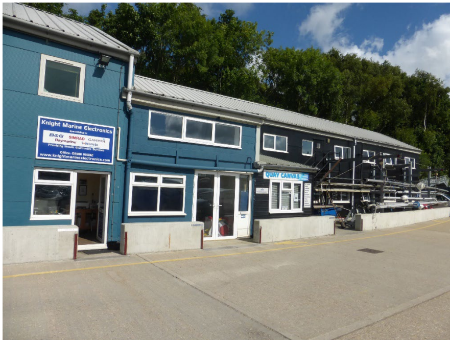
Existing Commercial Building
