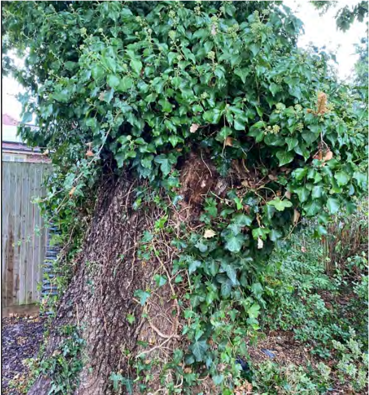
Photographic plate showing the stem of T1 with the ivy cladding partially removed to reveal a large historic pruning wound to the east.
