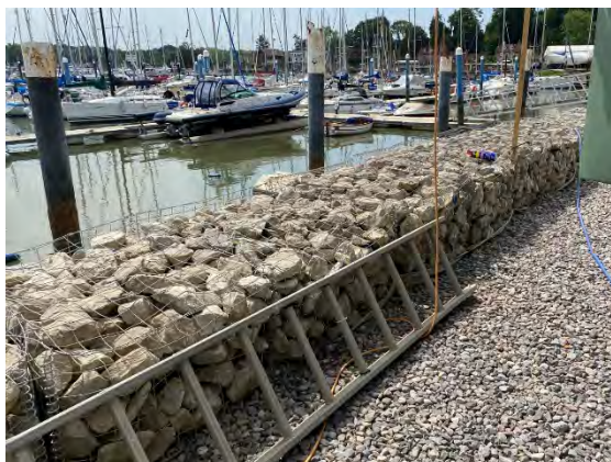
Photo 9: Recently installed Gabion Wall located along the central southern boundary. Note: these are not flood defences, they were installed to slow erosion
