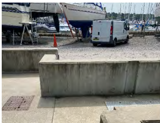
Photo 13: View of Permanent Concrete Flood Protection Measures
