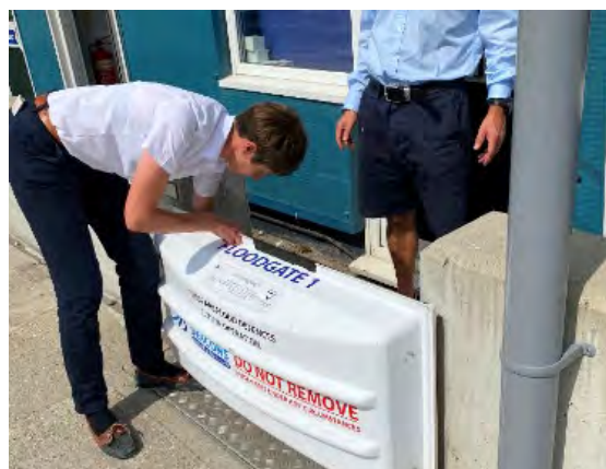
Photo 14: View of Demountable Flood Barrier
