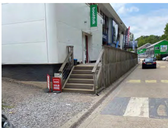
Photo 3: View of Deacons House, note the raised floor level, approx. 1.m elevation from ground level
