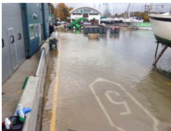
Photo 13: Water being held back by flood defences from The Workshops
