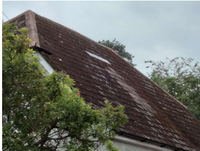
Photograph 6: North roof elevation of B1.
