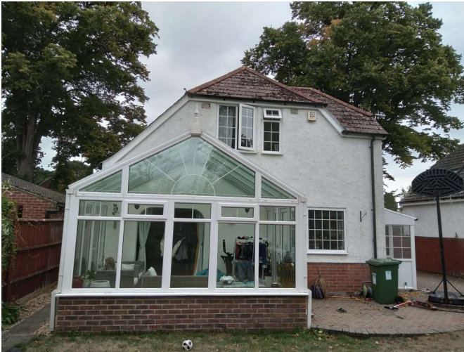
Photograph 3: West elevation of B1.
