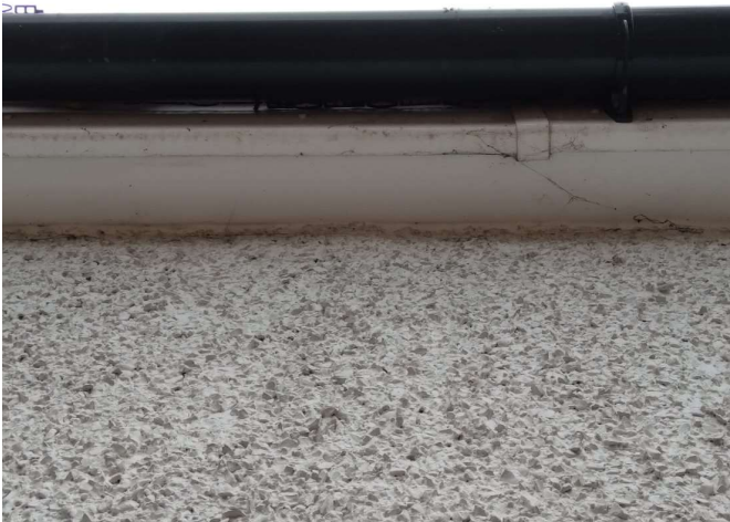
Photograph 5: North elevation of B1.
