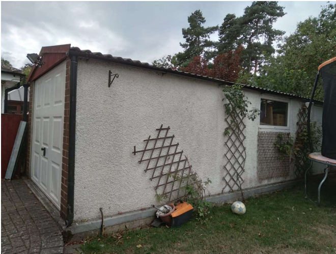
Photograph 9: East and south elevations of B2.
