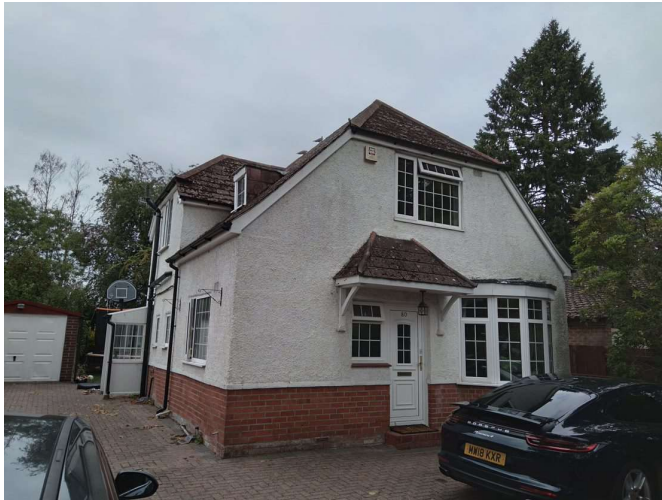
Photograph 1: East elevation of B1.
