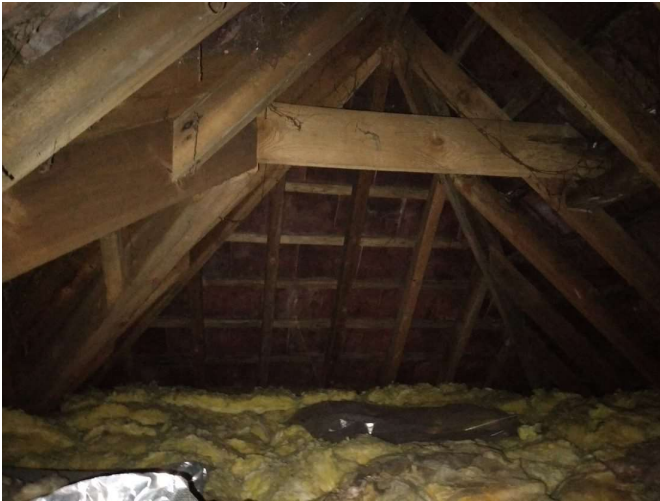
Photograph 7: Loft space within B1.
