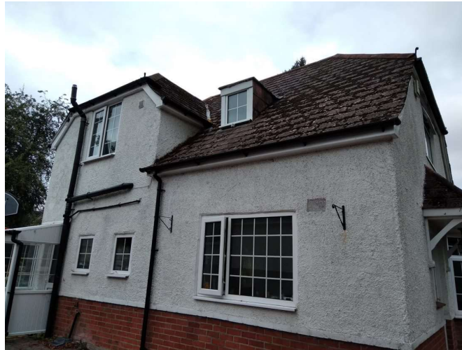
Photograph 2: South elevation of B1.
