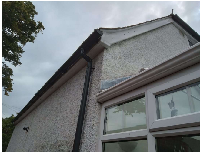
Photograph 4: North elevation of B1.
