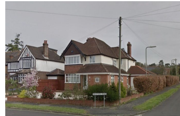
Fig.11 – 136 Western Road – timber clad gable over large bay window
