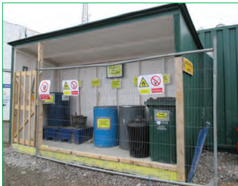
Figure 4.49 Dedicated hazardous waste storage area (courtesy J Murphy and Sons Ltd)
