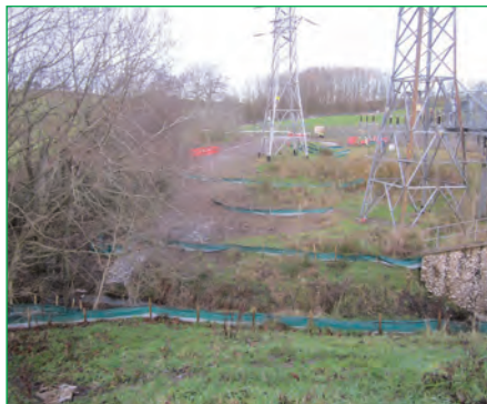
Figure 4.59 Silt fencing
