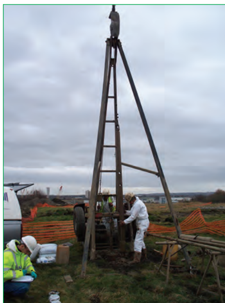
Figure 4.25 Soil testing being undertaken (courtesy Parsons Brinckerhoff)
