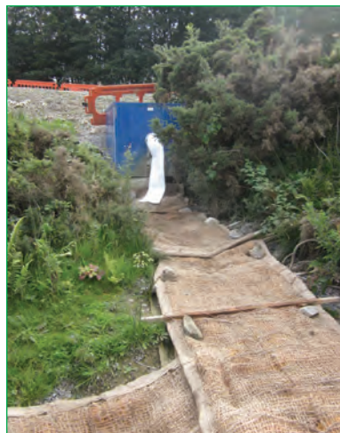
Figure 4.58 Dirt box, silt sock and sedimats
