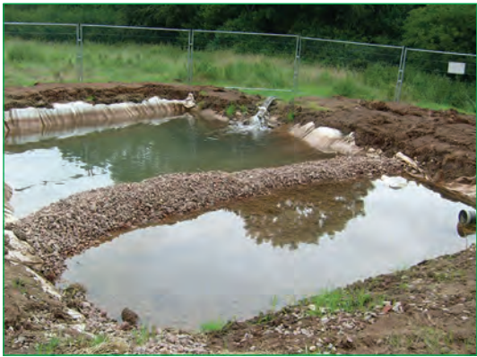
Figure 4.64 Settlement lagoon (courtesy Galliford Try plc)
