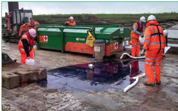
Figure 3.3 Spill drill training (courtesy BAM Nuttall)
