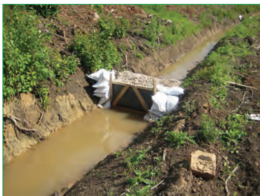
Figure 4.57 Silt fence (courtesy Galliford Try plc)
