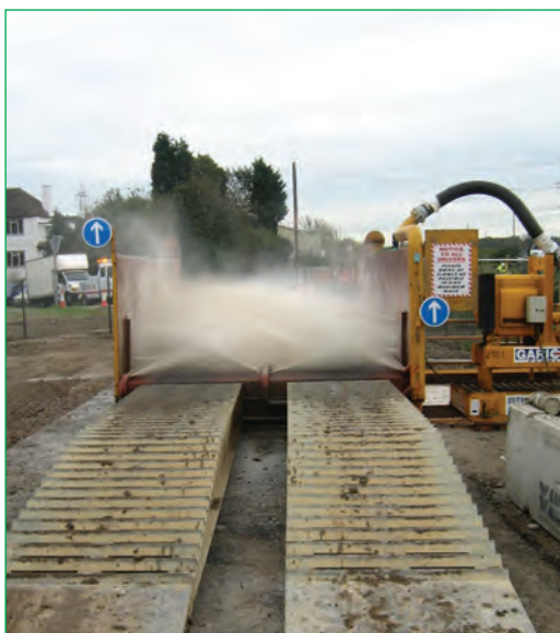
Figure 3.7 Wheel wash facility (courtesy Skanska)
