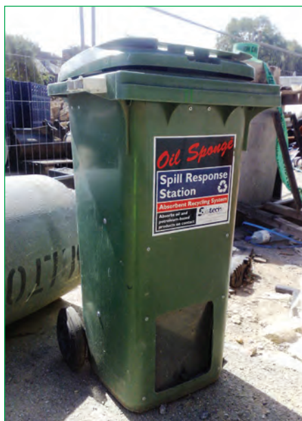
Figure 3.12 Spill response station (courtesy BAM Nuttall)
