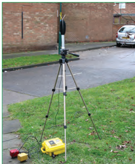
Figure 4.35 Free-field noise monitoring equipment (courtesy Parsons Brinckerhoff)
