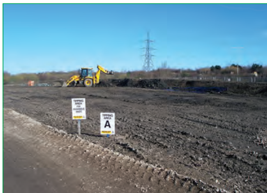
Figure 4.27 Land remediation (courtesy Parsons Brinckerhoff)
