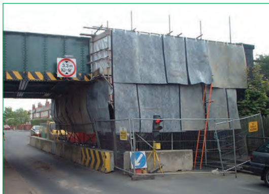
Figure 4.32 Acoustic screening (courtesy BAM Nuttall)
