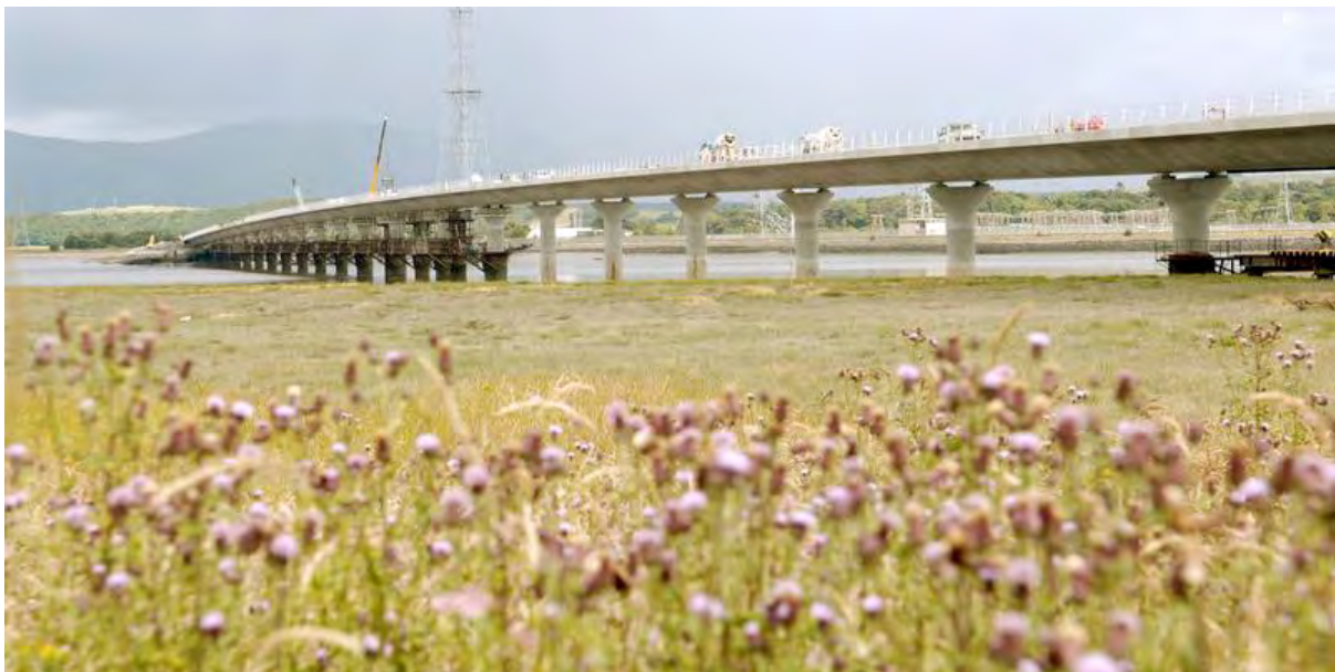
Bridge maintenance (courtesy of SEPA)
