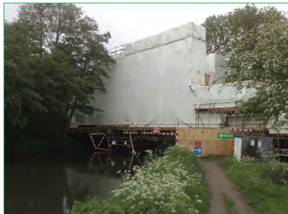
Figure 4.66 Encapsulation of blasting works (courtesy BAM Nuttall)
