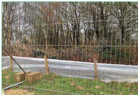
Figure 4.14 Great crested newt fencing (courtesy Brookfield Multiplex)
