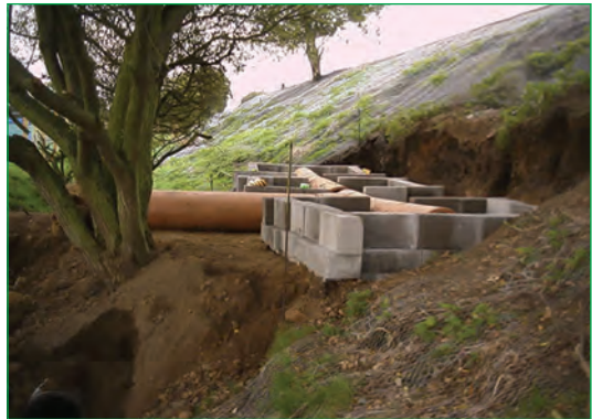
Figure 4.9 Badger sett construction (courtesy BAM Nuttall)
