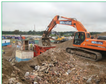
Figure 4.42 On site crusher (courtesy Skanska)
