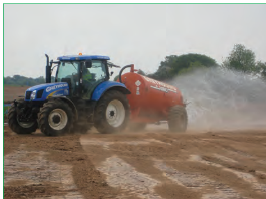
Figure 4.29 Dust suppression (courtesy Galliford Try plc)
