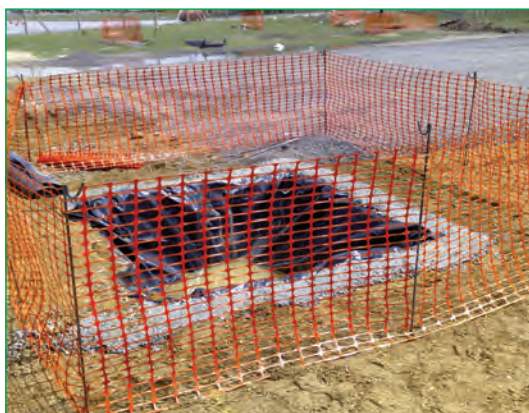
Figure 4.61 Lined washout pit (courtesy BAM Nuttall)
