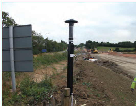
Figure 4.31 Dust monitoring (courtesy Balfour Beatty)
