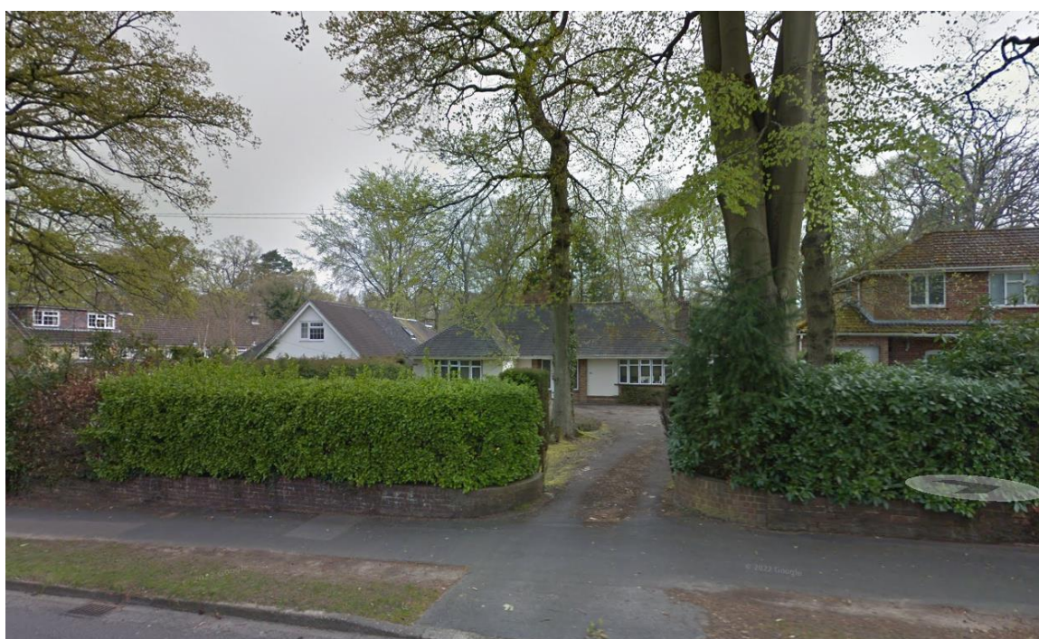
No. 92 as it appeared previously in 2015 (when it was single storey)
