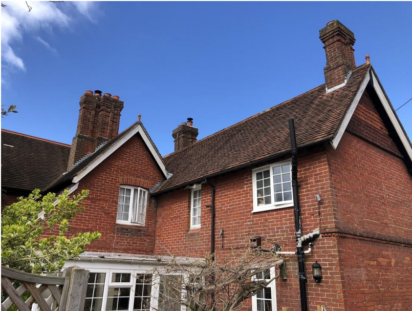
5.13. Rear elevation and east gable of application site.
