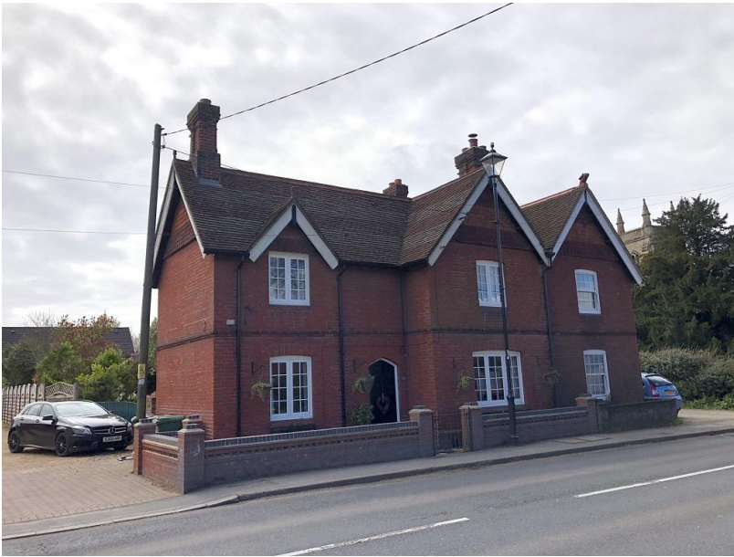
5.01. Front elevation to the High Street with no. 45 on the right hand side.
