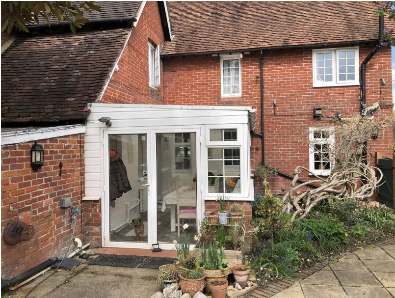
5.14. Rear of application site 1.
