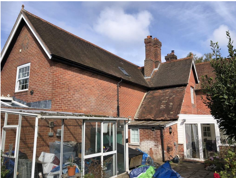
5.11. Adjoining property 45 High Street on left hand side, lean-to and small gable to application site.
