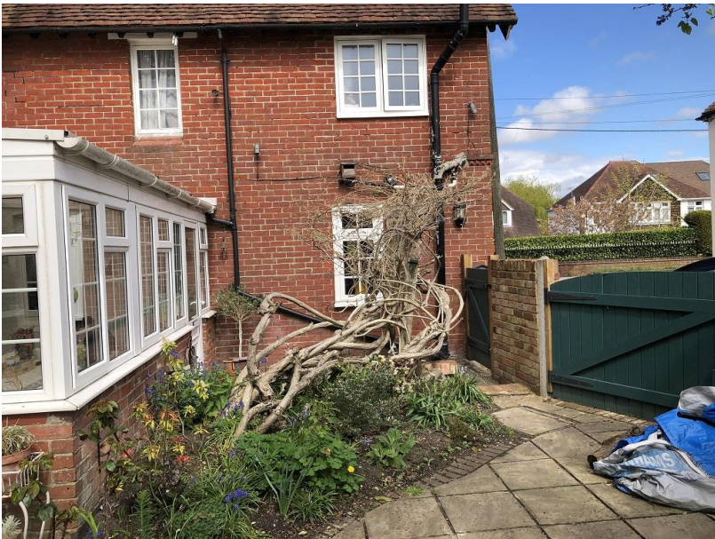
5.15. Rear of application site 2.
