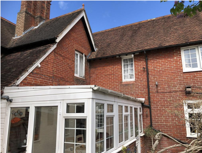
5.16. Rear of application site 3.
