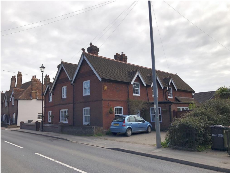
5.04. Adjoining property no. 45 viewed from the High Street.
