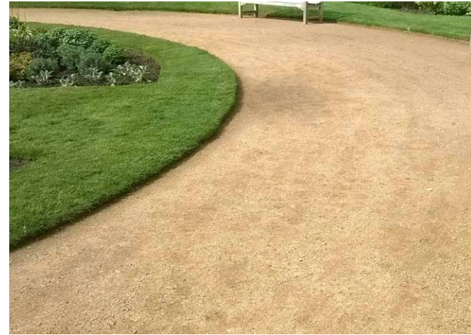
Self binding gravels - Hoggins drive surface
