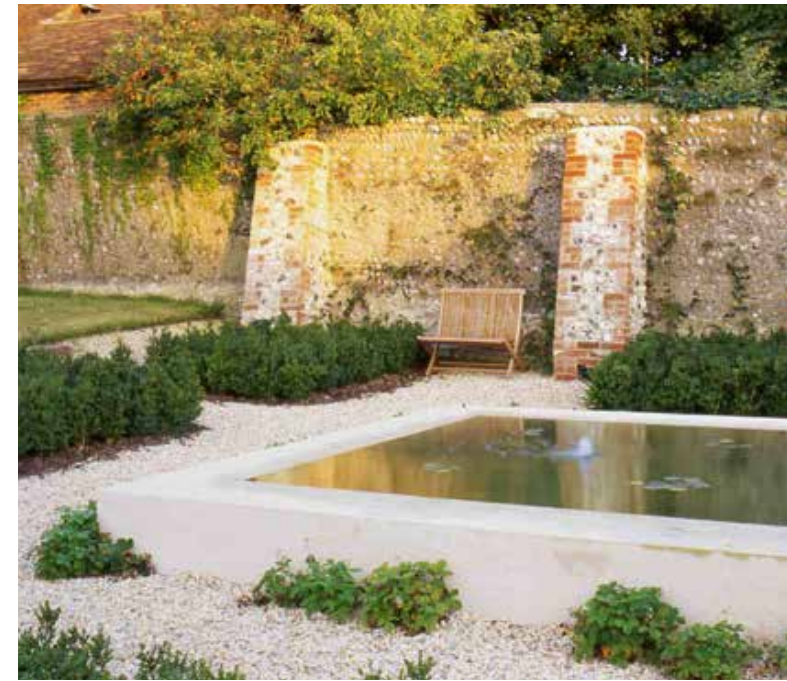
South facing productive wall built from brick and flint
