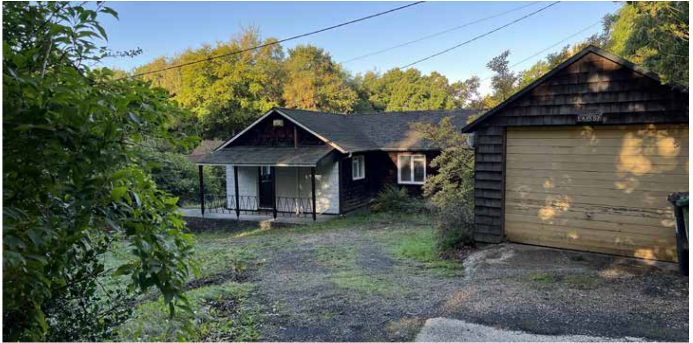
Larkby seen from Kew Lane, looking westwards
