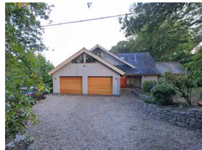
Neighbouring property to the north of Larkby
