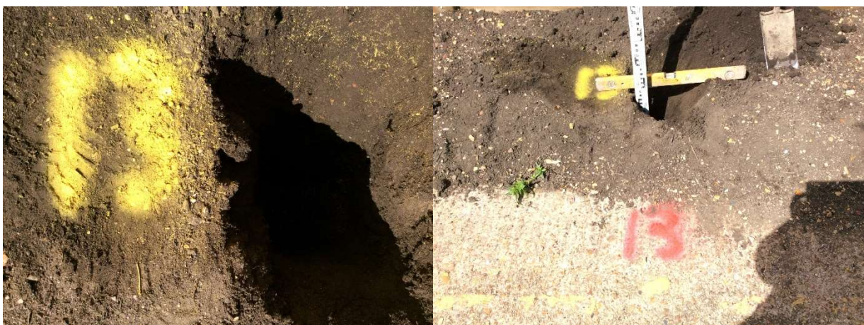
Photographs 3a & 3b - Hand Pit 13 in the Soft Landscaping
