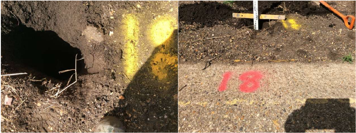
Photographs 4a & 4b - Hand Pit 18 in the Soft Landscaping
