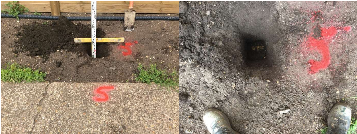
Photographs 1a & 1b - Hand Pit 5 in the Soft Landscaping
