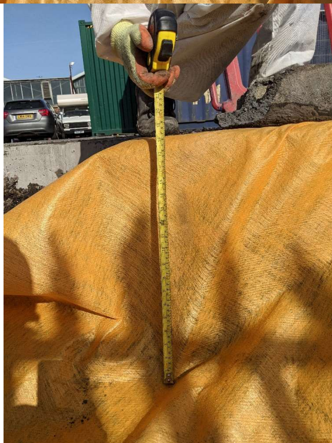
Photographa 8a & 8b - Installation of geotextile membrane under the soft landscaping.
