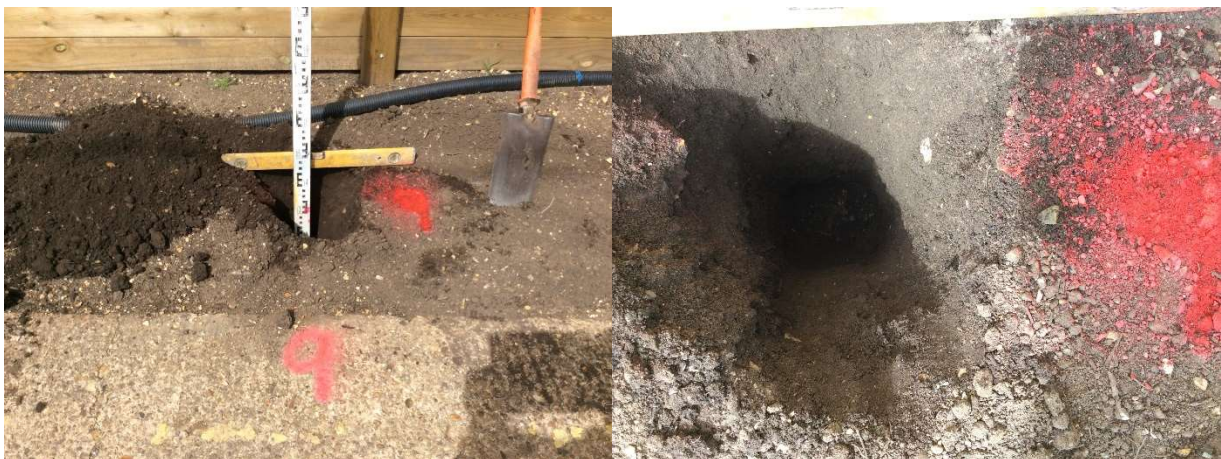
Photographs 2a & 2b - Hand Pit 9 in the Soft Landscaping
