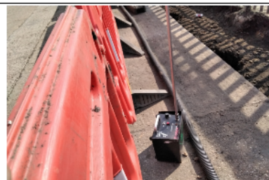
West boundary line location C WSS013 25.03.22 12.37
