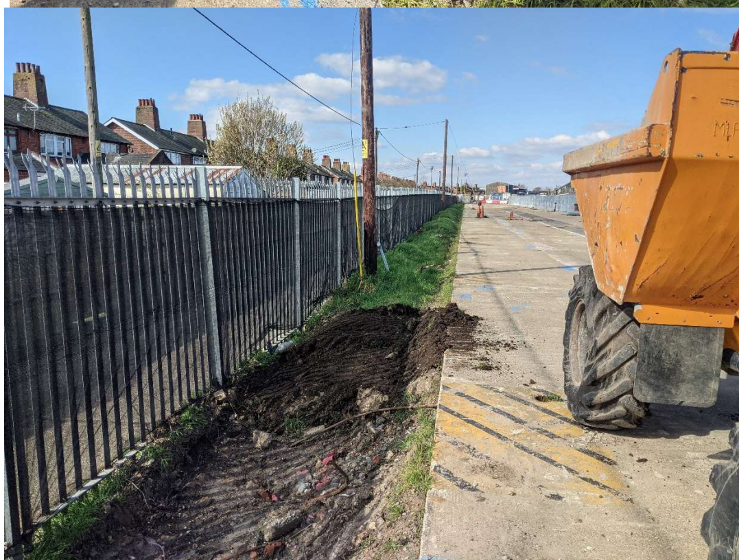
Photographs 7a & 7b - Excavation of previous Soft Landscaping -
