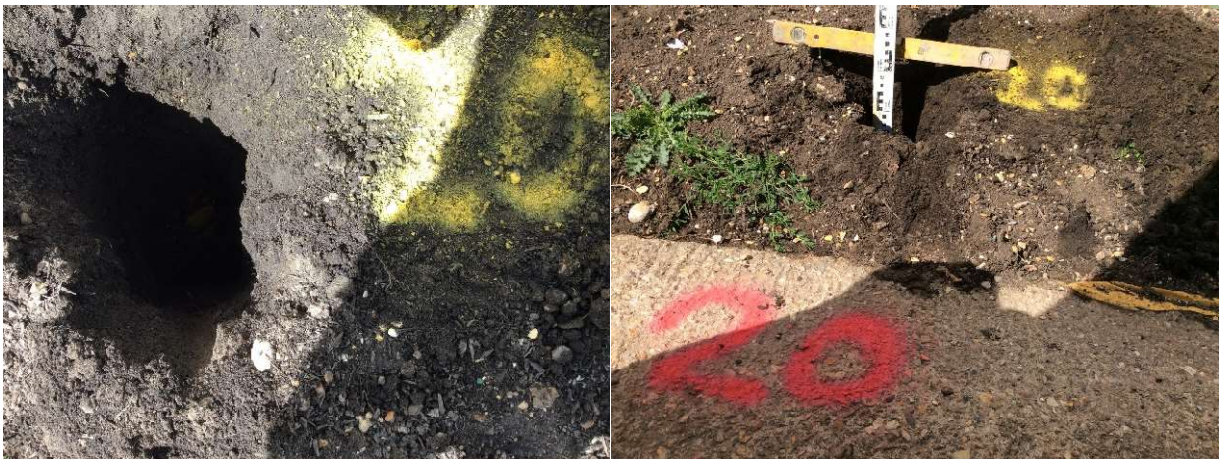
Photograph 5a & 5b - Hand Pit 20 in the Soft Landscaping
