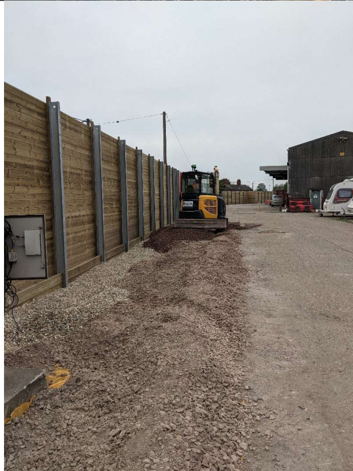
Photographs 6a & 6b - Soft Landscaping finish on the inside of the acoustic fence.
