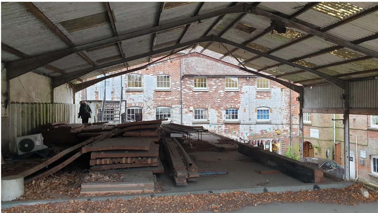
View of void over existing shop units, with the Mill building in the background and retaining wall to the left.
