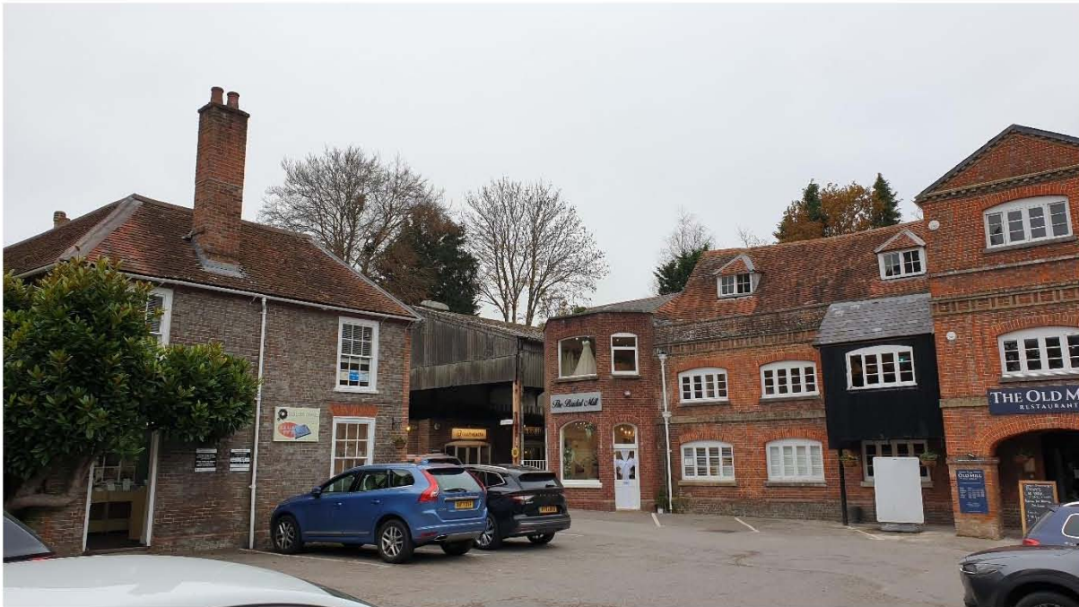
View from front of site, with main Mill building to the right, Mill House to the left and the existing canopy in the background
