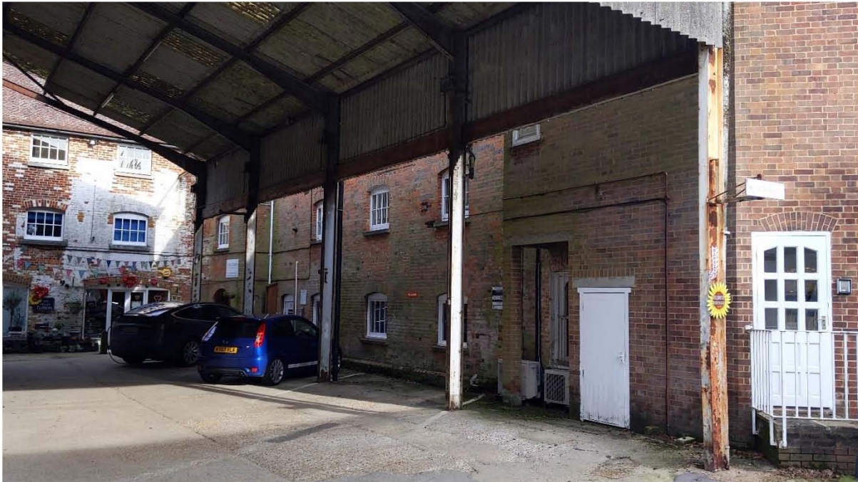
View under the canopy of the main Mill building
