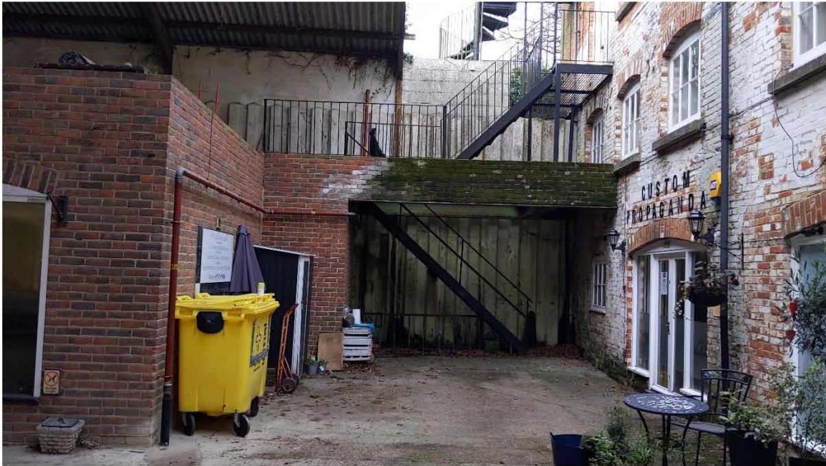
The existing fire escape staircase
