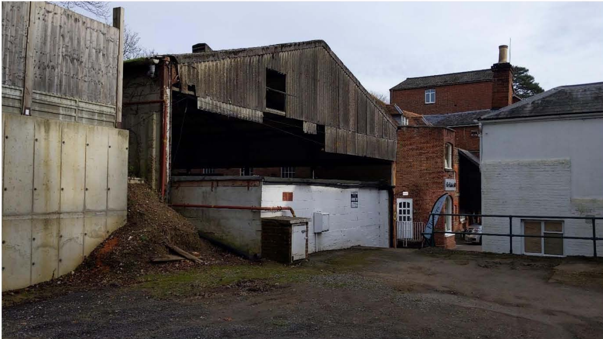
View of canopy from higher ground level. Retaining wall visible in left of photo
