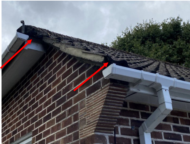
Figure 10. Gap present in the mortar (taken September 2022)
