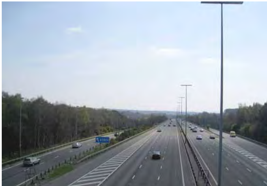
Figure 30. M27 motorway near Netley Hill
