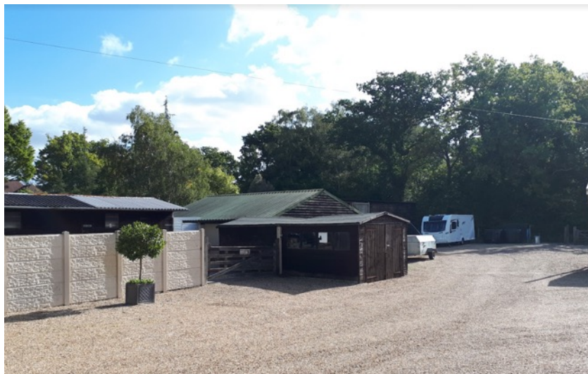
Figure 7. Outbuildings along the eastern boundary of the site (taken October 2022).
