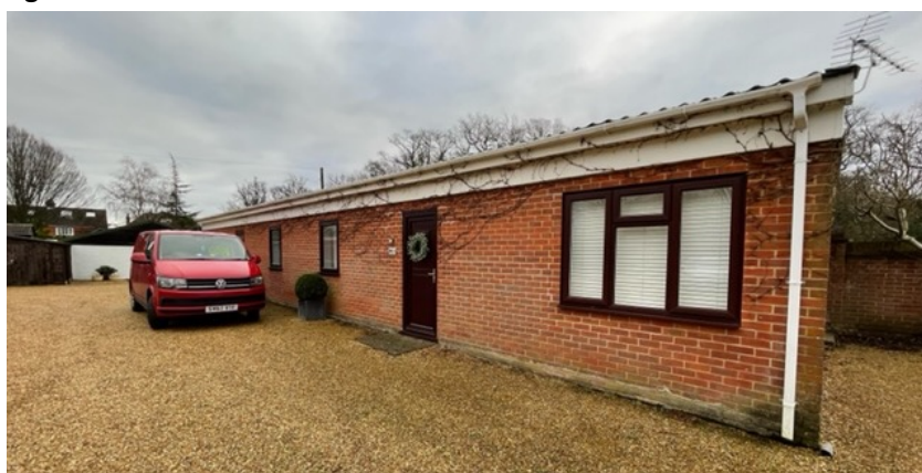
Figure 8. View of the annex on site
