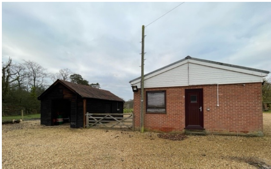
Figure 6. Annex building (right) and adjacent outbuilding to the south, view from eastern aspect
