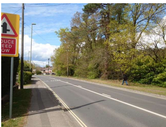
Photograph 3: Existing Conditions on Moorhill Road (A27) Northbound
