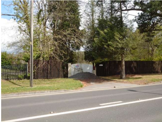
Photograph 1: Existing Northern Site Access Conditions
