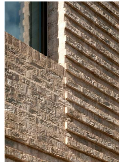
Brick detail, decorative projecting brickwork
