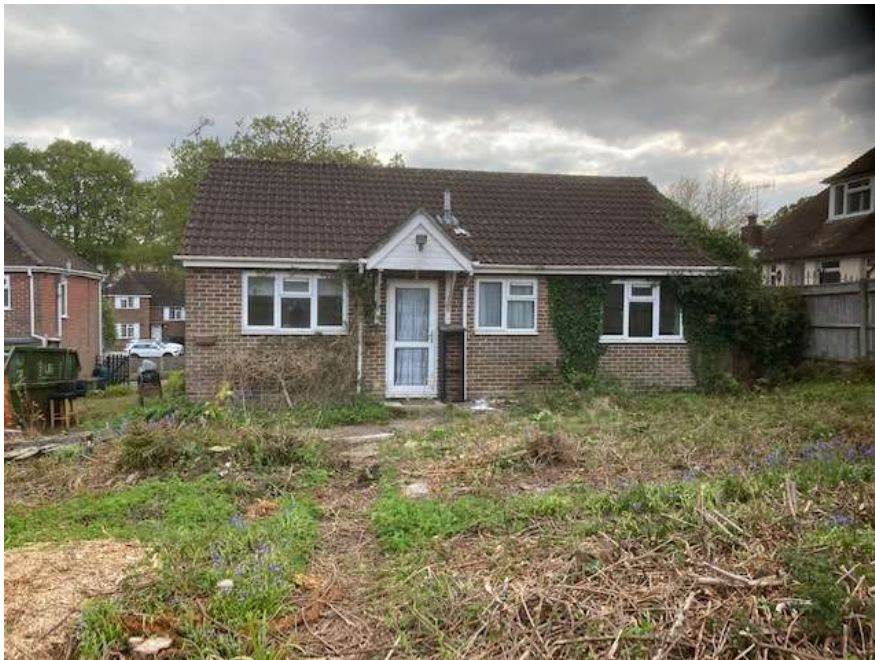
Fig.5 – Photograph showing the rear (north) elevation of the existing bungalow at 242 Leigh Road.
