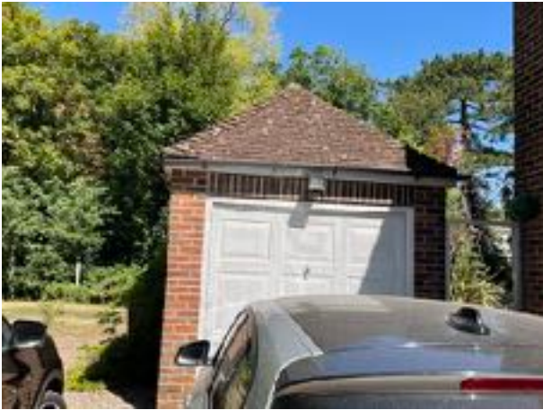
Figure 7 - South elevation of garage
