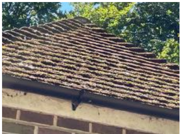
Figure 12 - No raised or missing tiles
