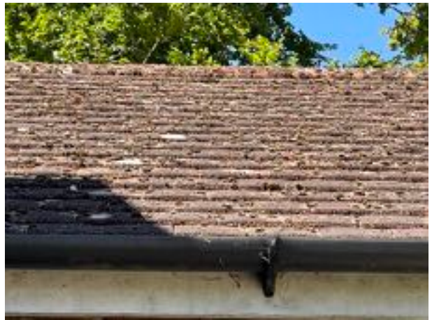
Figure 10 - No raised or missing tiles
