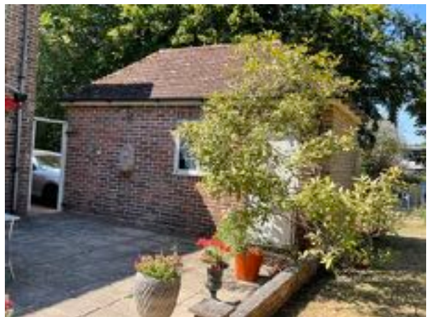
Figure 6 - East elevation of garage
