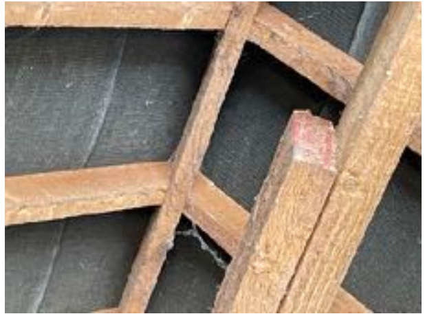
Figure 8 - Cobwebs at ridge, No gaps between rafters
