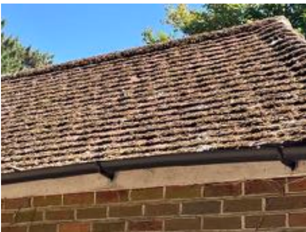
Figure 11 - No raised or missing tiles
