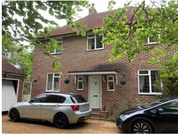
Figure 11 West elevation of existing house and garage
