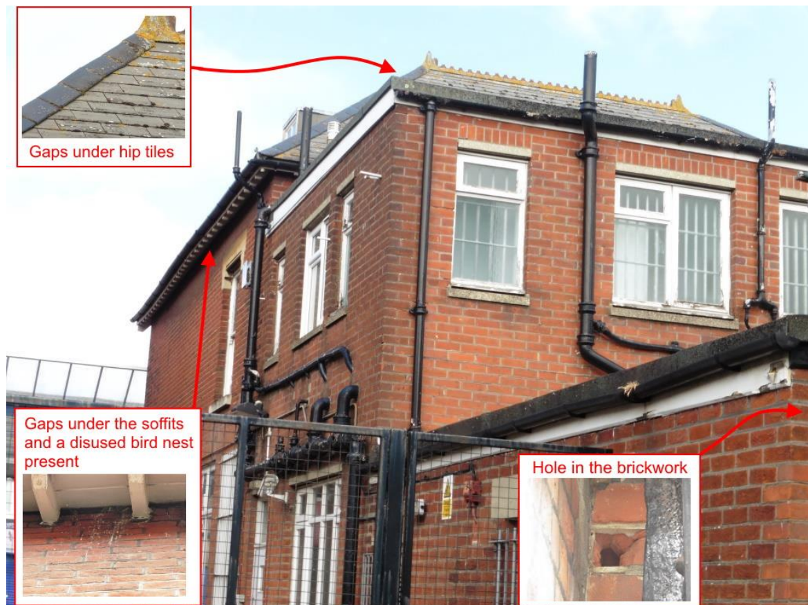
Image 4.3.1.2. Location of bat access points on the south & east elevation of the Post Office.
