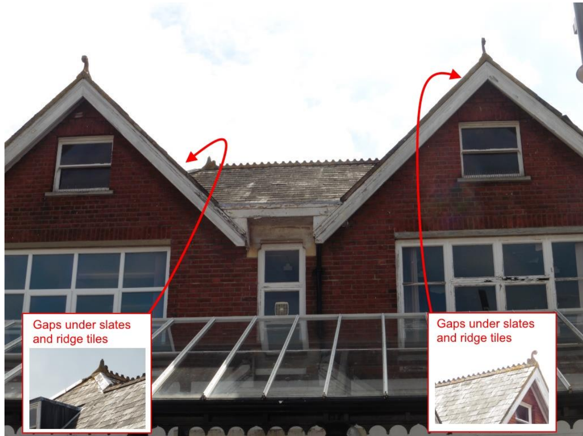
Image 4.3.1.1. Location of bat access points on the west elevation of the Post Office.
