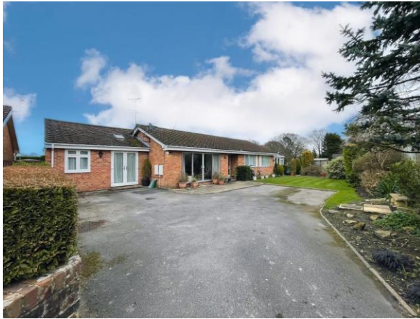
Front elevation from south west
