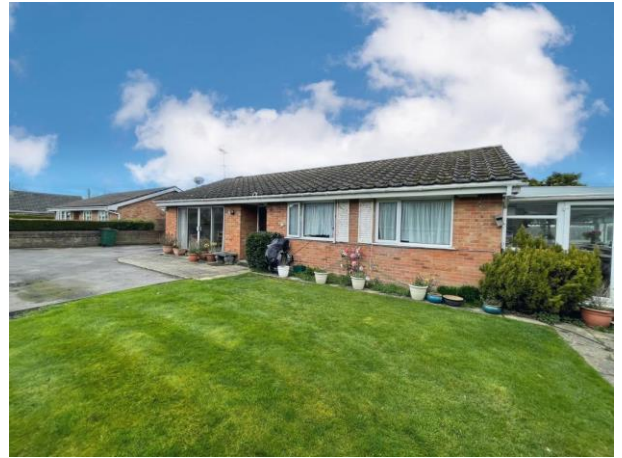
Front Elevation from south east
