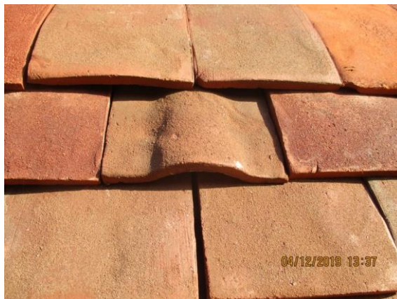
Image 5.6.2.1. Examples of a Bat Access Tile and a Bat Access Slate.
