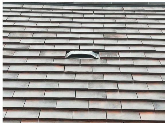
Image 5.6.2.1. Examples of a Bat Access Tile and a Bat Access Slate.
