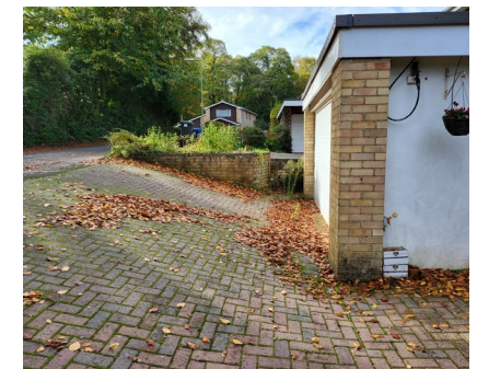
Photographs of existing steep driveway
