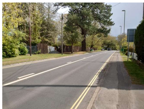
Photograph 4: Existing Conditions on Moorhill Road (A27) Southbound
