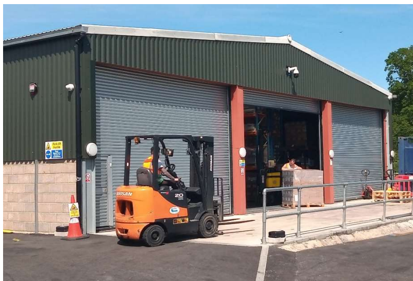
Above - Photo showing the front of existing Building 1.
