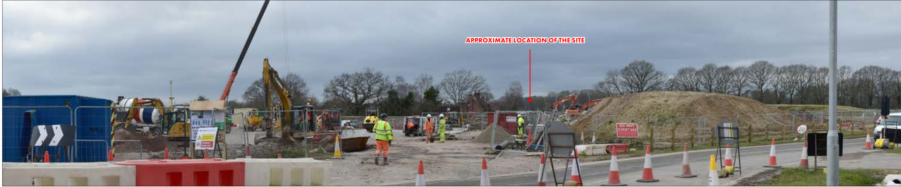
PHOTOGRAPH – VIEWPOINT 6 VALUE: MEDIUM VIEW LOOKING SOUTH-EAST FROM NORTHERN SECTION OF WOODHOUSE LANE LOOKING ACROSS THE ROAD. THE FOREGROUND OF THIS VIEW COMPRISES CONSTRUCTION OPERATIONS AND MATERIAL STOCK PILING. VIEWS OF THE SITE ARE TRUNCATED DUE TO THE COMBINATION OF THE CONSTRUCTION ACTIVITIES AND THE LAYERS OF VEGETATION.
