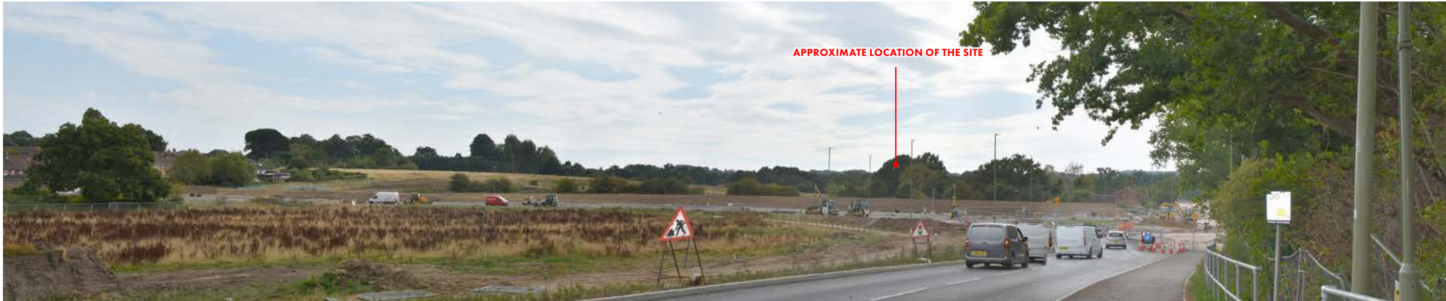
PHOTOGRAPH – VIEWPOINT 18 VALUE: MEDIUM VIEW LOOKING SOUTH-WEST FROM THE NORTHERN TIP OF WOODHOUSE LANE. THE PYLONS ARE APPARENT, BUT VIEWS OF THE SITE ARE TRUNCATED DUE TO THE COMBINATION OF TOPOGRAPHY AND THE LAYERS OF VEGETATION.
