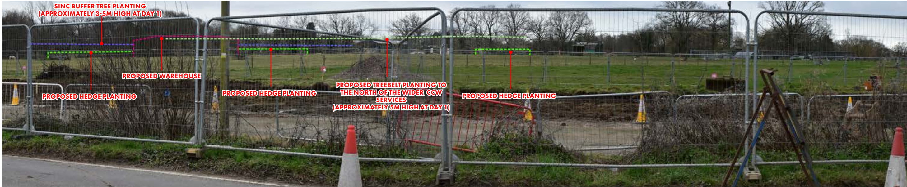
VIEWPOINT 2 - YEAR 1 AFTER COMPLETION
