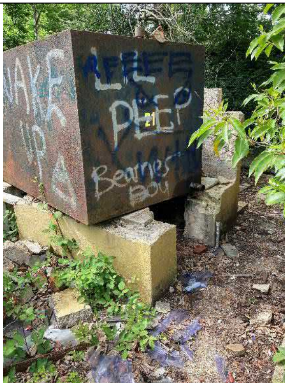
Photograph 5- Rusted Green tank in the northeast of the site. Facing North
